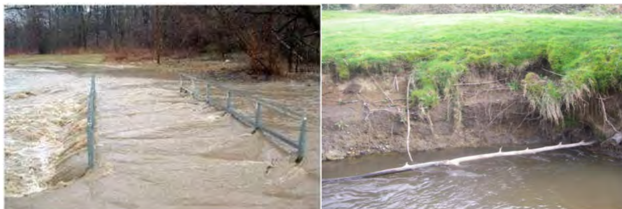
Figure 4-4: Examples of Flooding and Erosion Impacts
