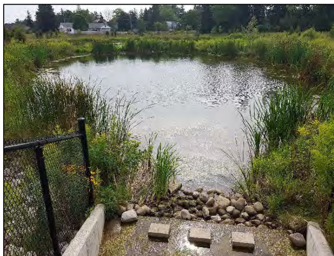
Figure 5-1: A wet pond SWM facility provides water quality treatment via the settlement of suspended pollutants and flood control via the temporary detention and peak flow reduction
