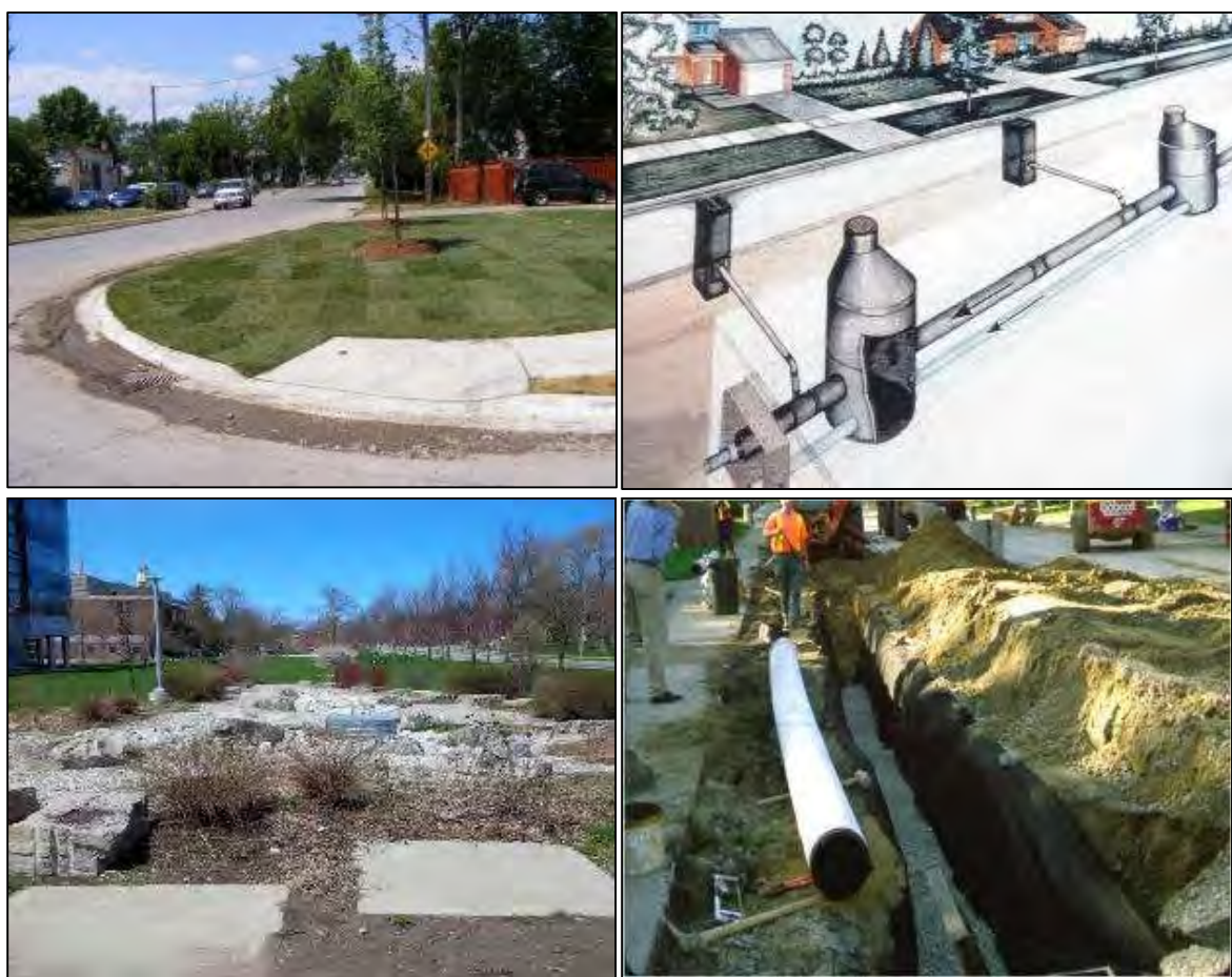
Figure 5-3: Example LID Practices from Top Left to Right: Soil Amendment (Mississauga, ON), Exfiltration System (Etobicoke ON); Exfiltration System (Guelph, ON); Perforated Pipe (Toronto, ON)
