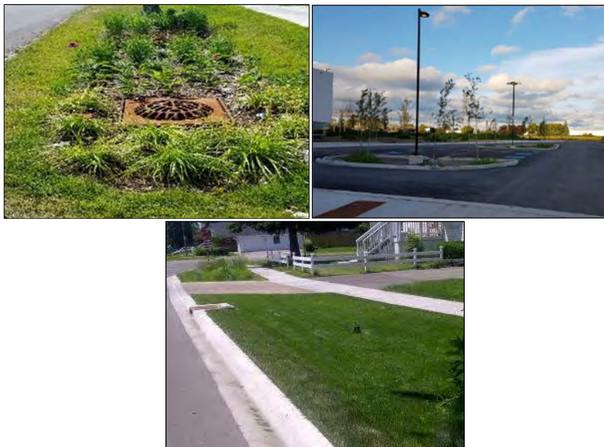
Figure 5-4: Example LID Practices from Top Left to Right: Bioretention (Toronto, ON); Bioretention (Bostwick Community Centre, London, ON); Grass Swale (Mississauga, ON)
