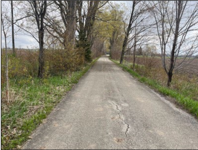
Image 5: Shows existing asphalt driveway.
