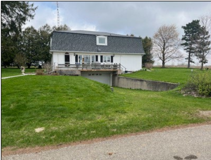
Image 12: Shows existing structure and conditions for test pit survey.
