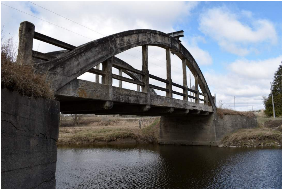
Figure 8: East side of Bridge 21-WG, looking northwest
