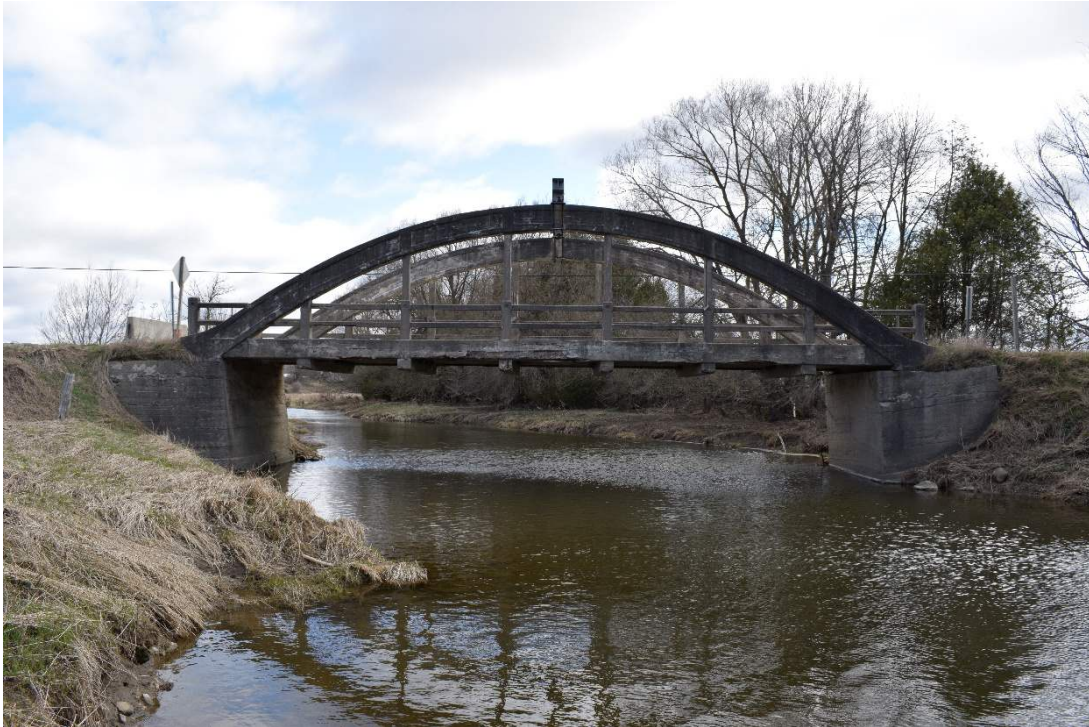
Figure 7: West side of Bridge 21-WG, looking east
