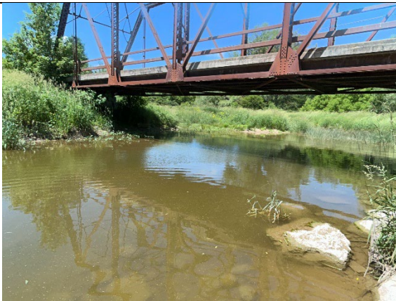
Photo 23: Inlet of the structure. Facing west.
