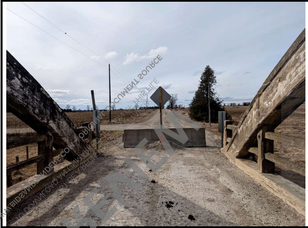
Photo 3 North approach from centre of structure
