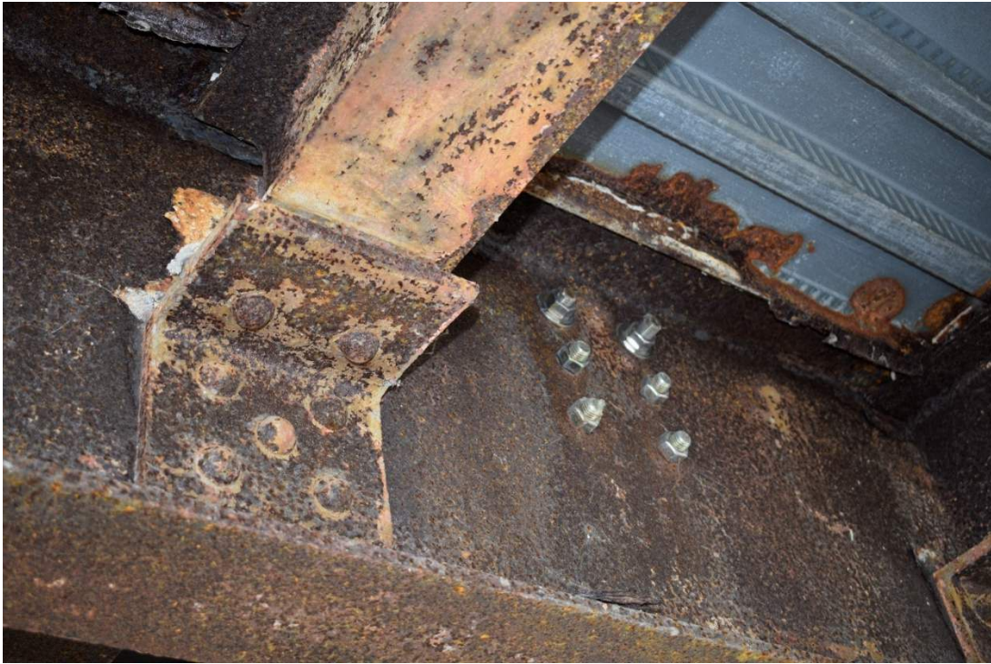
Figure 53: Example of original riveted construction and later bolt and nut repair
