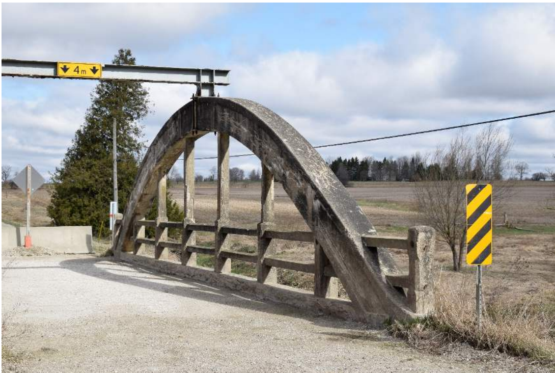
Figure 12: Eastern arch of Bridge 21-WG
