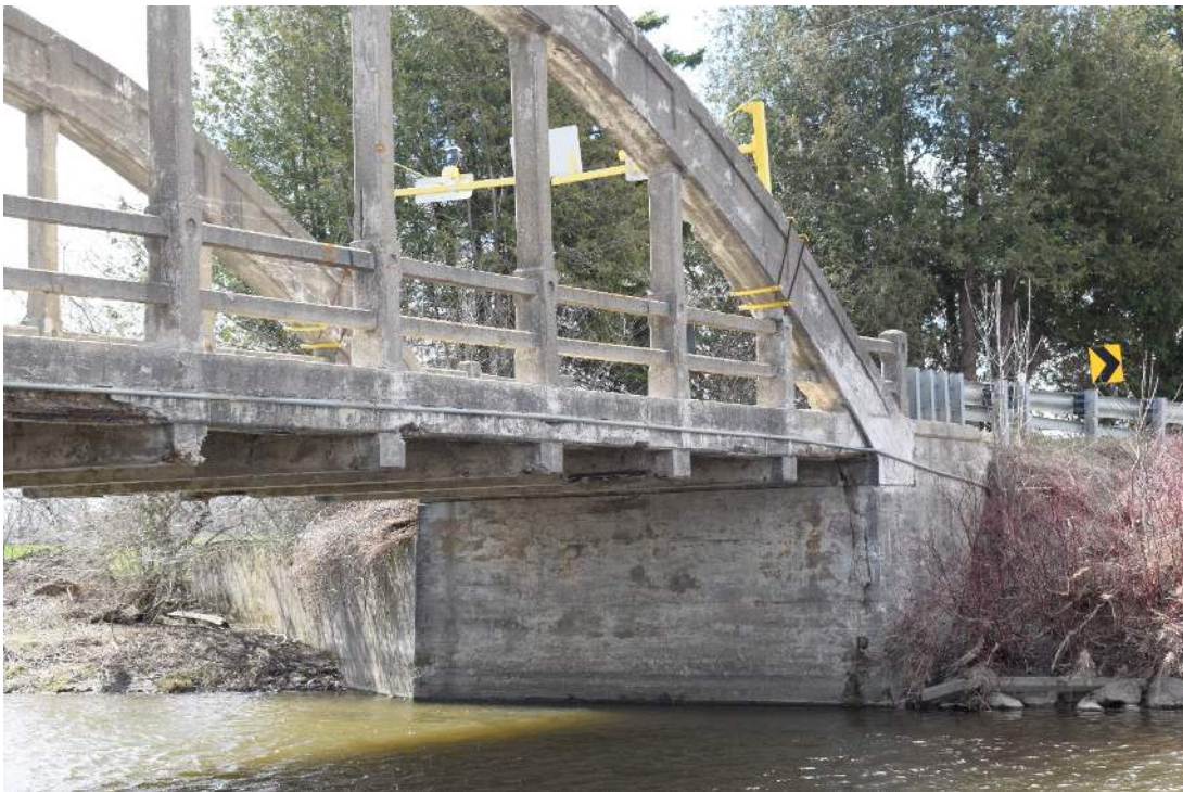
Figure 33: West bridge abutment
