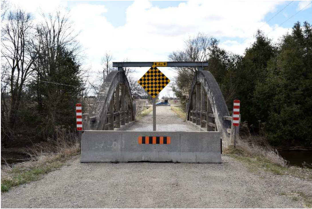
Figure 9: Northern approach to Bridge 21-WG, looking south
