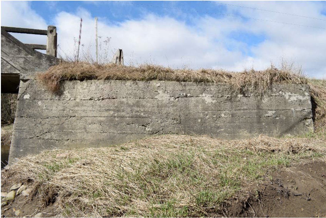
Figure 15: Typical example of abutment wing, note visible impressions of planking used in the forming process and the separations between lifts of concrete
