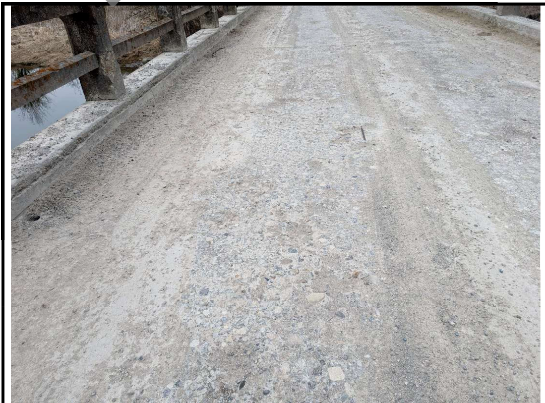
Photo 10 Moderate to severe scaling on deck wearing surface
