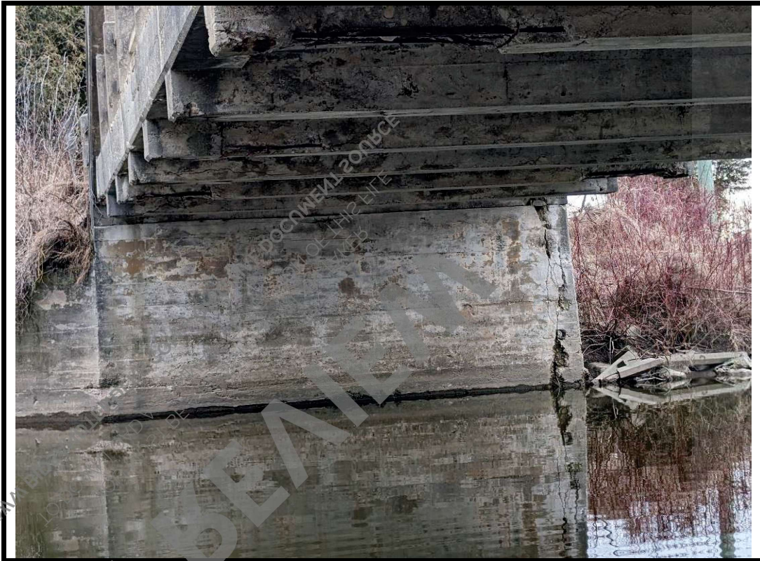
Photo 13 Wide crack on north corner of east abutment wall
