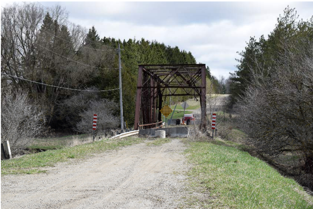
Figure 40: Eastern approach to Bridge 30-WG
