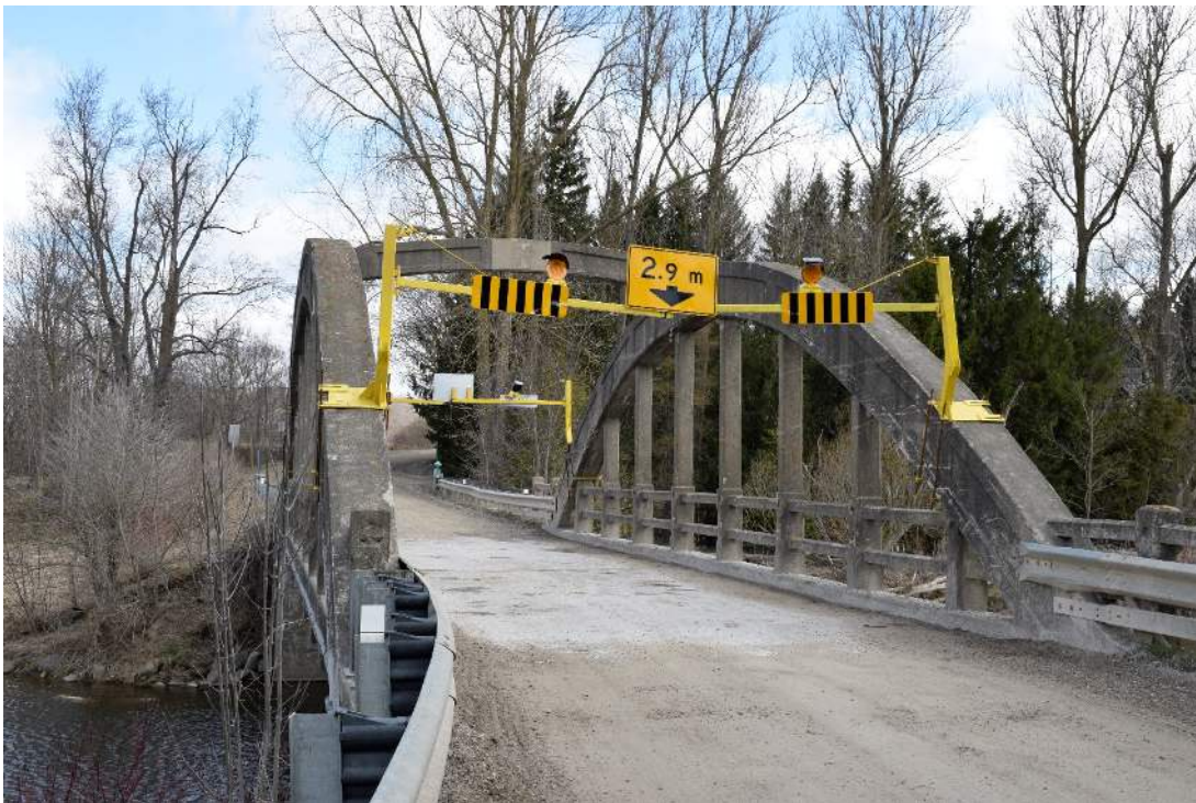
Figure 29: West approach to Bridge 29-WG
