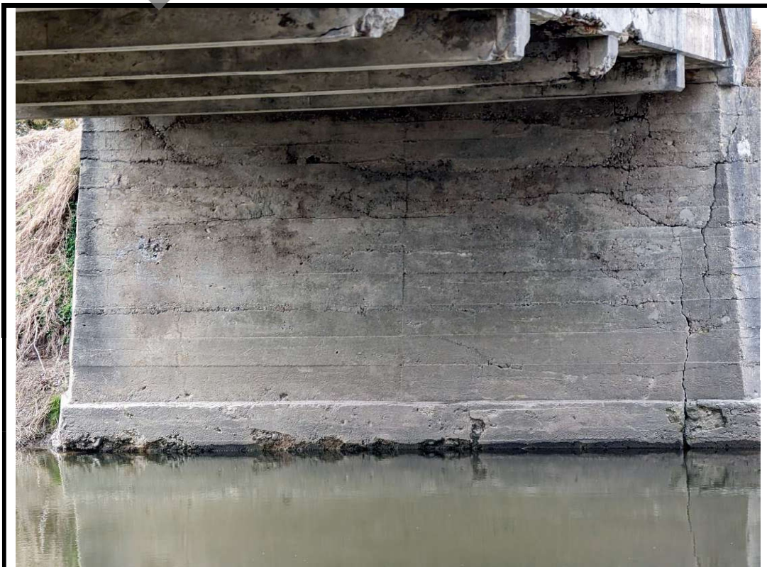
Photo 12 Erosion and wide cracks noted at north abutment.
