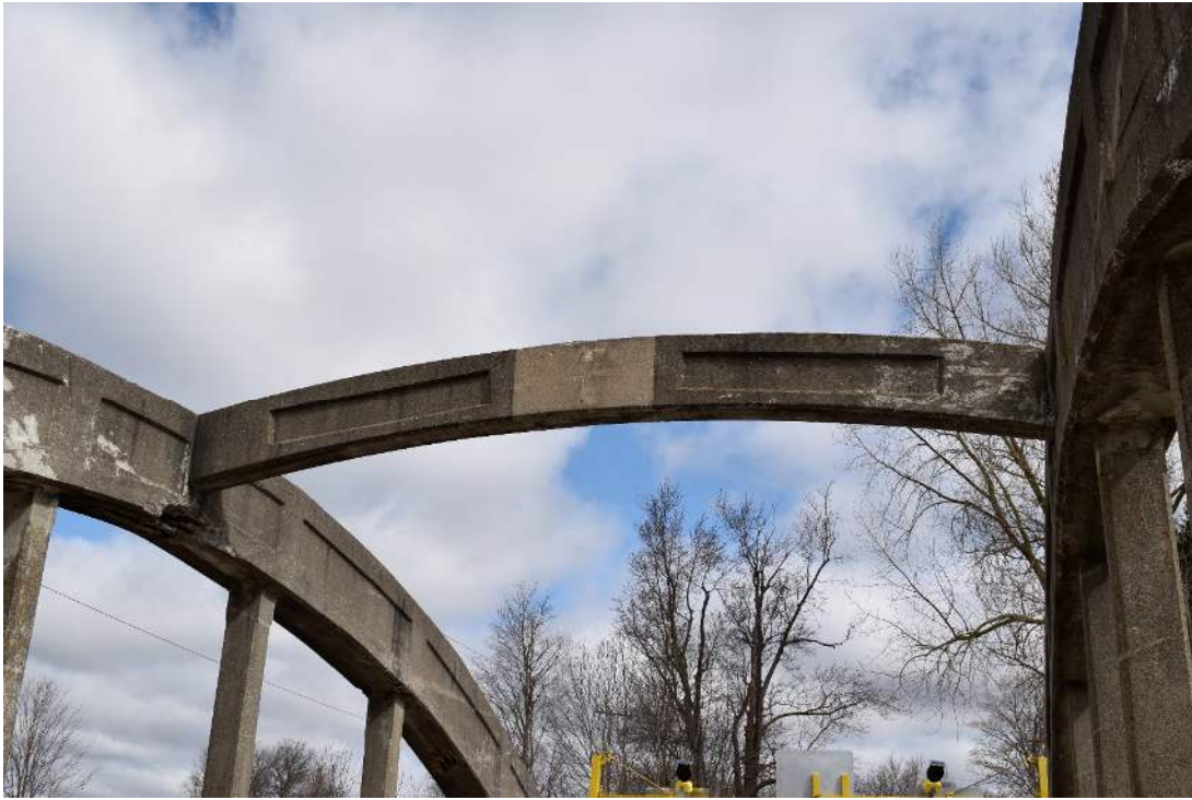
Figure 34: Original cast concrete tie beam
