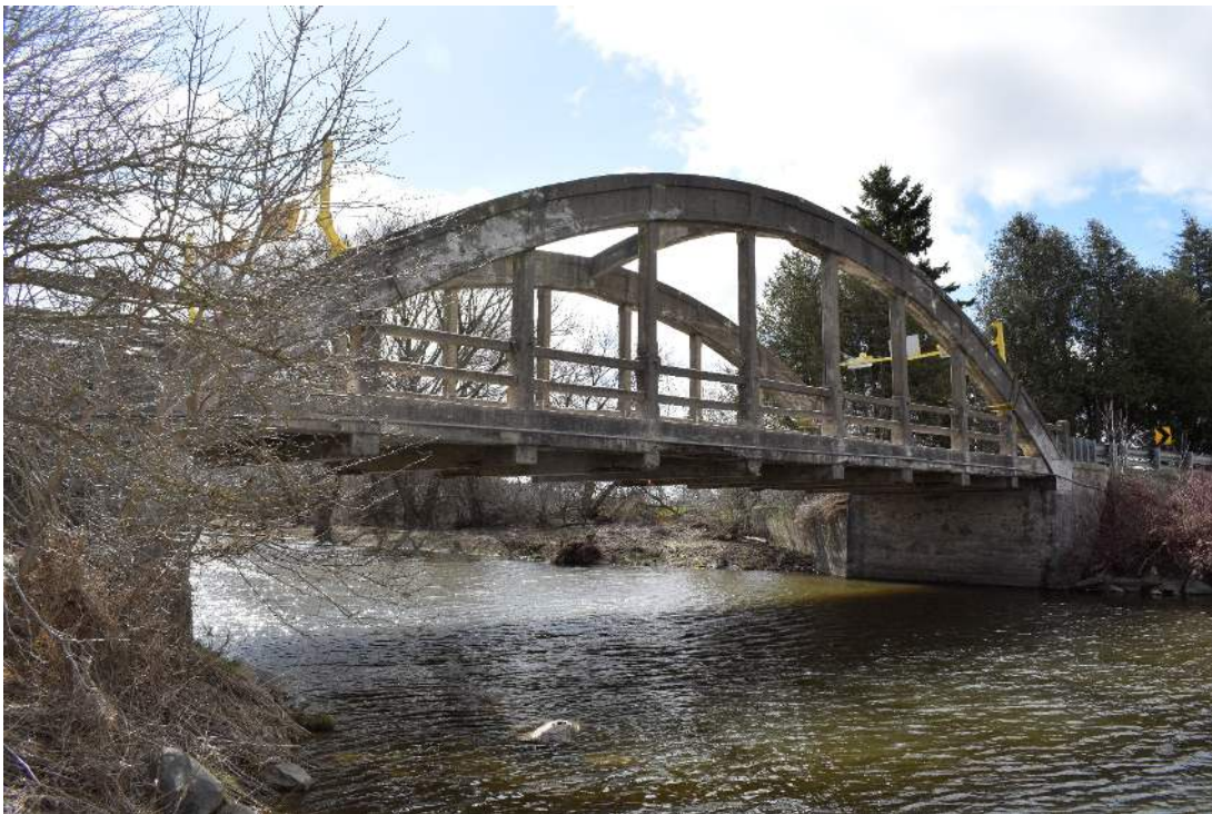
Figure 27: North side of Bridge 29-WG
