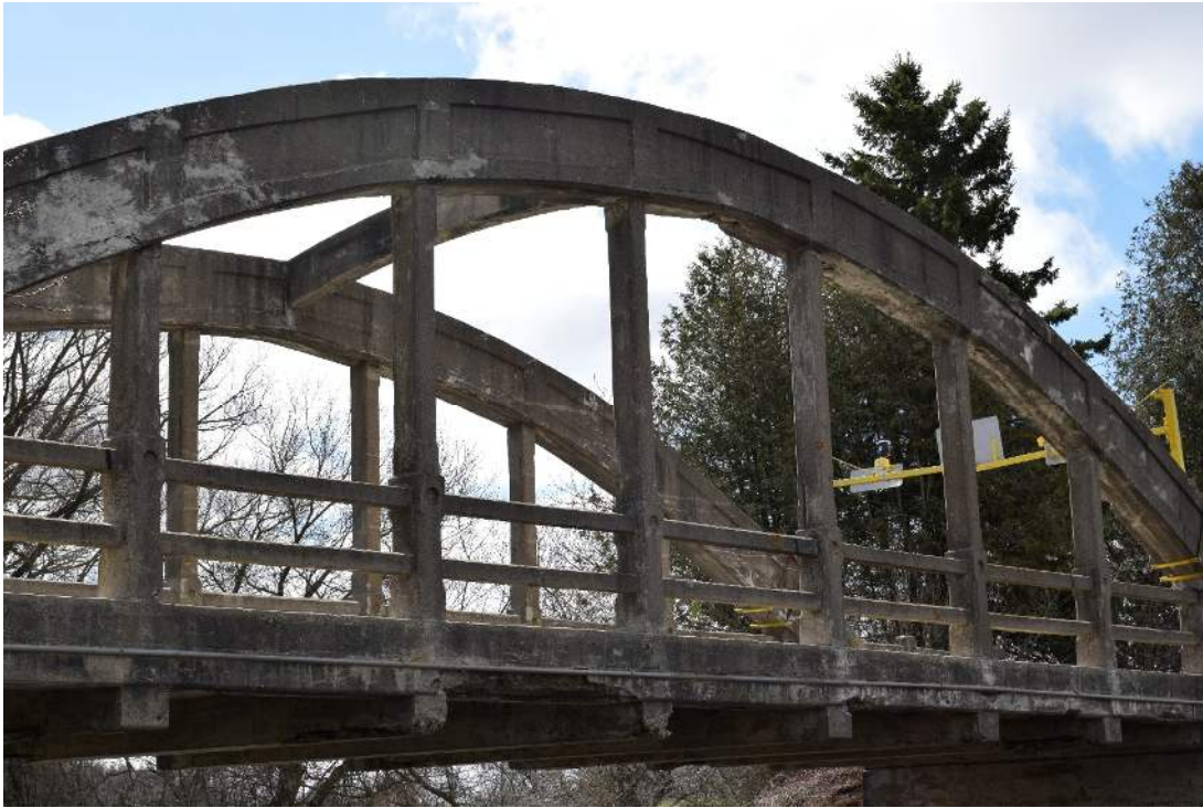
Figure 36: Focus on detail cast into arch and associated supports and guardrail, exterior of north side
