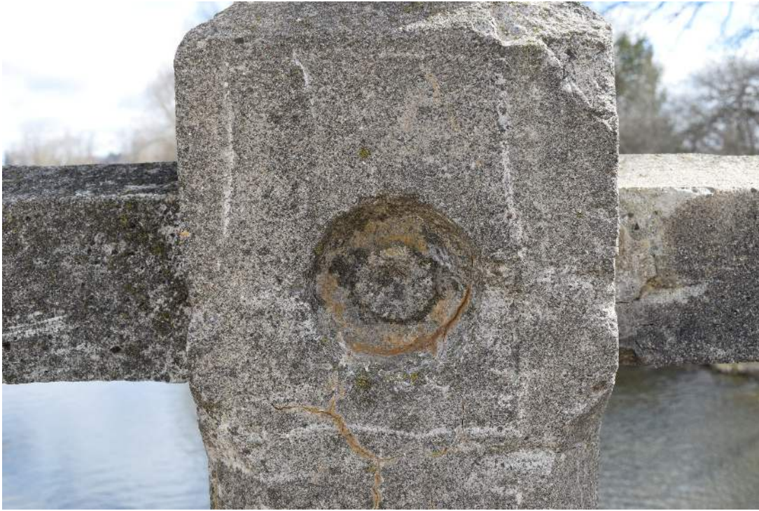
Figure 19: Close up of typical recessed 'florete' cast into guard rail supports
