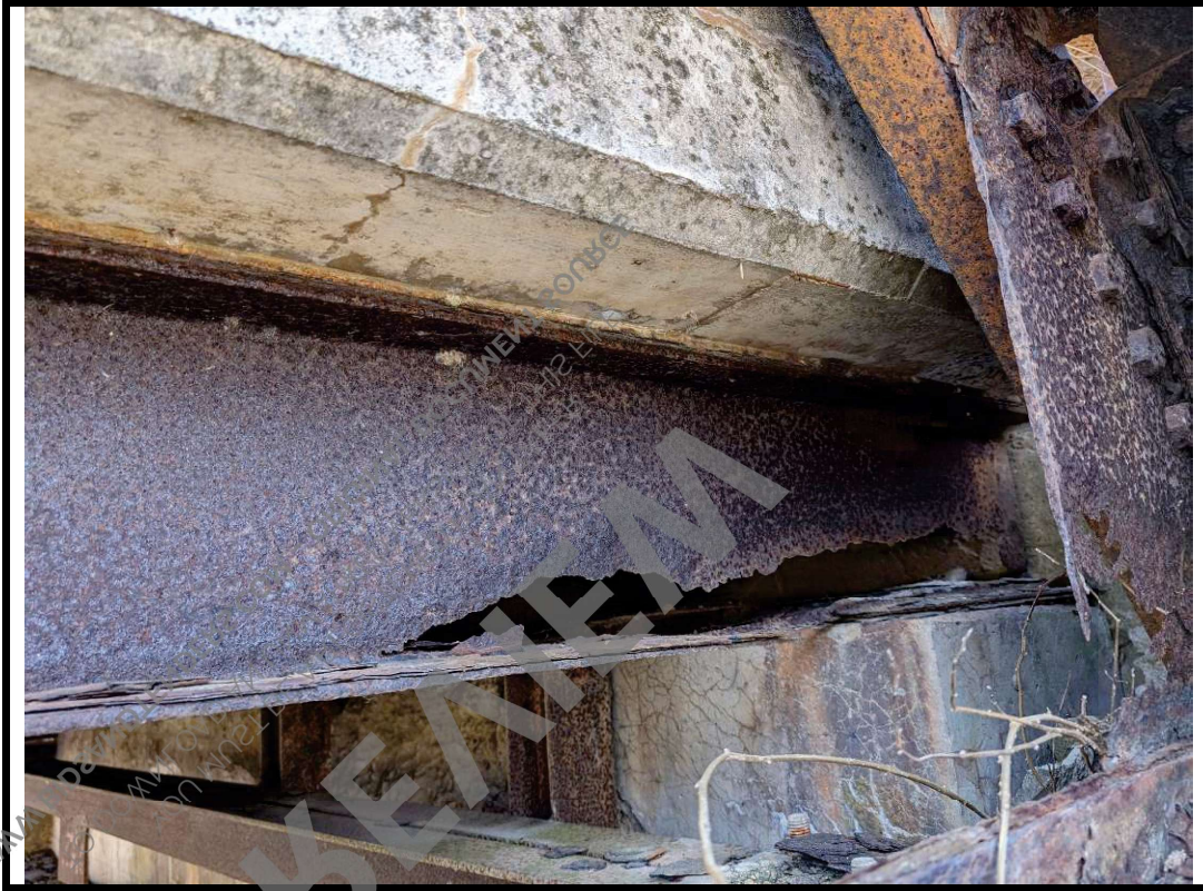
Photo 11 Perforations at girder ends at the east side of structure
