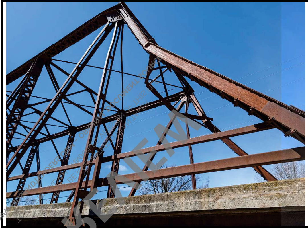
Photo 9 Deformation of truss elements and bracing at east side of structure
