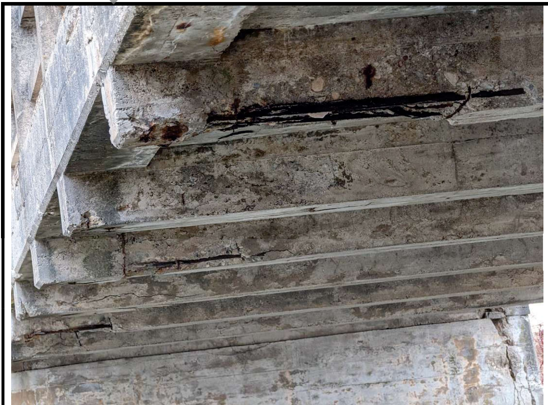
Photo 12 Spall with exposed corroded reinforcement on floor beams and soffit exterior
