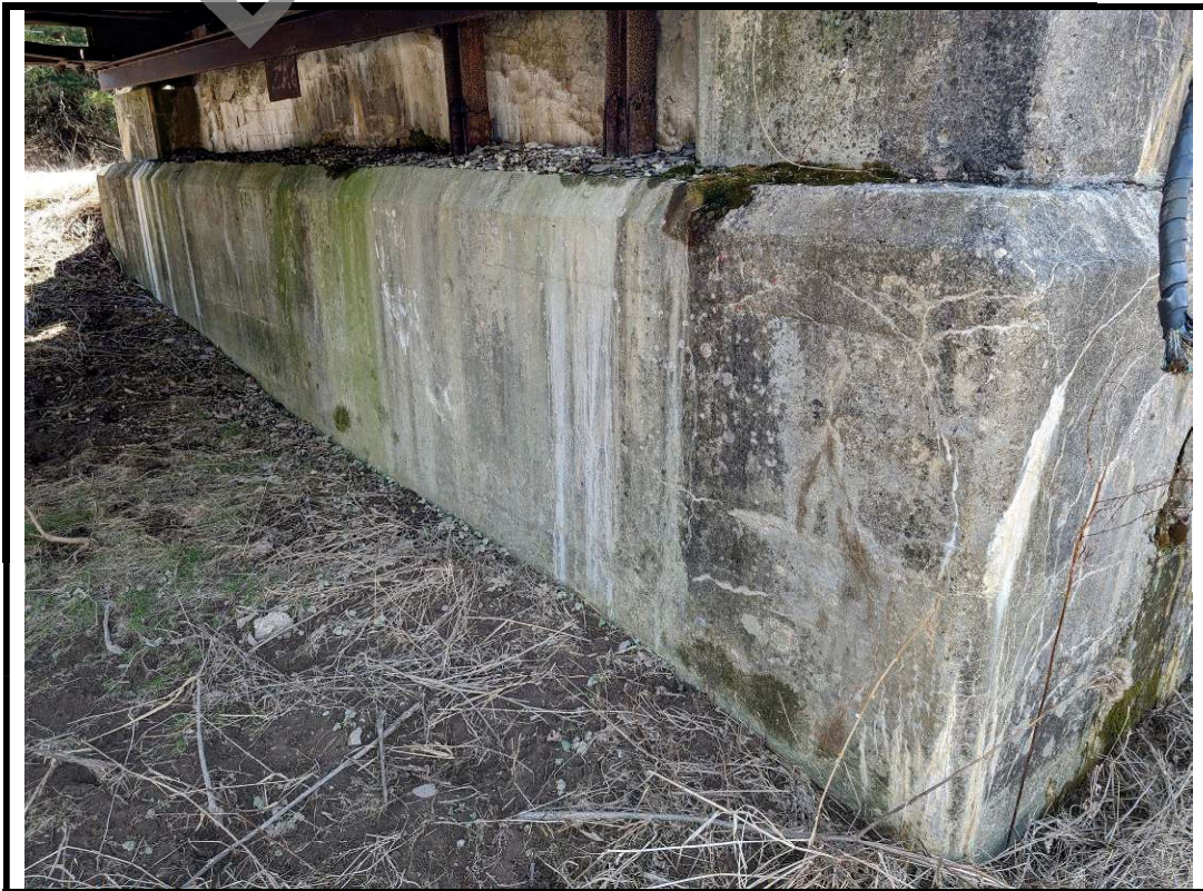
Photo 14 Concrete Disintegration, Scaling, and Cracks at east abutment wall
