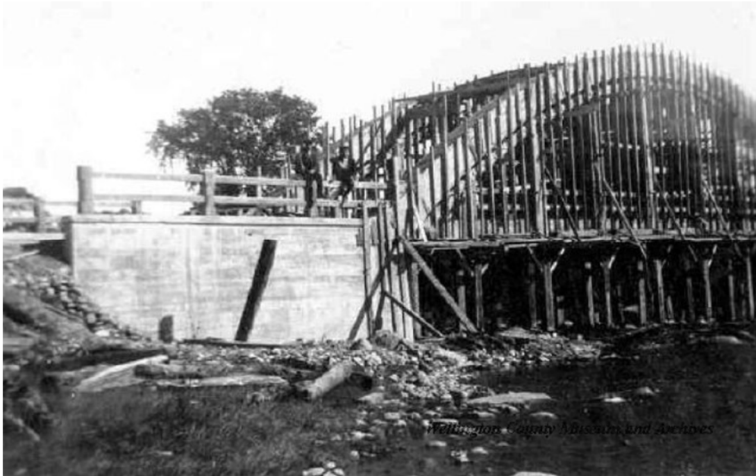
Figure 3: Undated historic image of the construction of a bowstring arch bridge, image 3032 of the Mattaini Fond on file with Wellington County Museum and Archives
