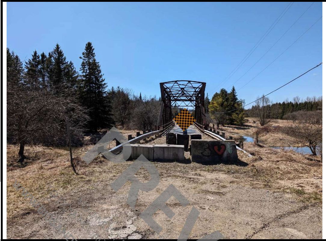
Photo 1 Structure from east approach
