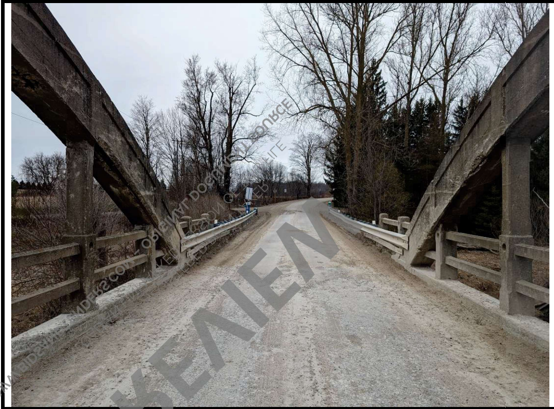
Photo 3 East approach from centre of structure
