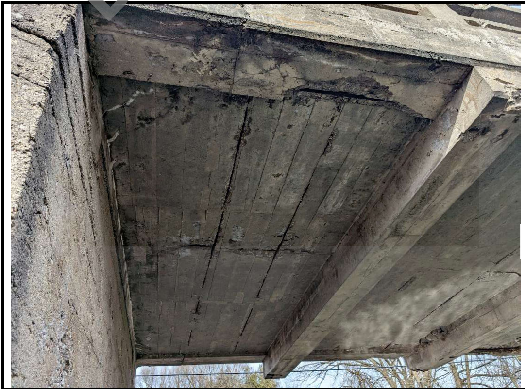
Photo 18 Delaminations, medium cracks with area of efflorescence and severe spalls with exposed corroded reinforcement noted soffit
