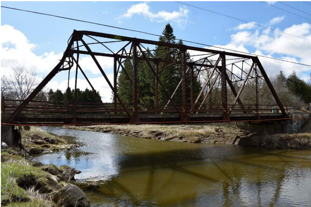
Figure 42: North side of Bridge 30-WG
