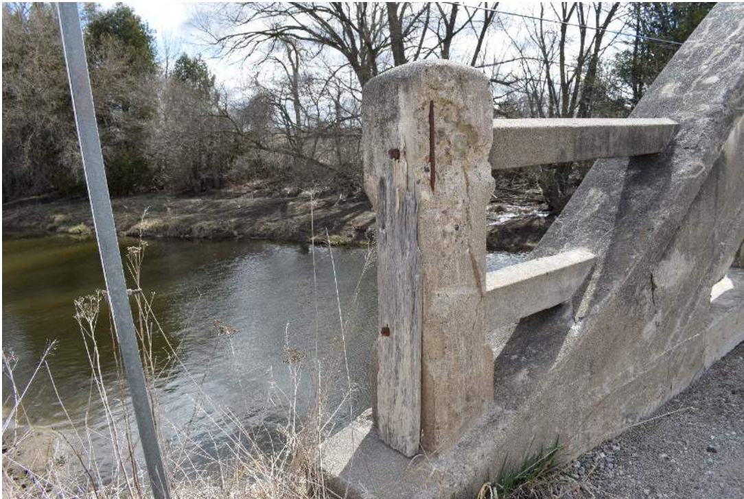
Figure 20: Example of concrete spalling revealing underlying steel reinforcement material
