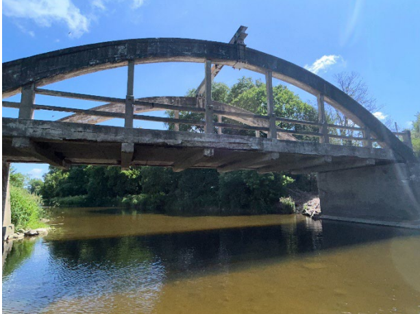
Photo 5 Outlet of bridge. Facing north.
