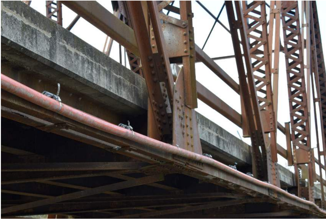
Figure 49: Example of original riveted construction
