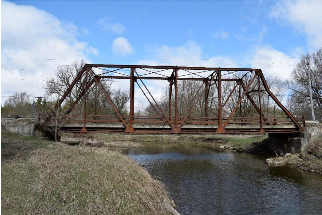
Figure 41: South side of Bridge 30-WG
