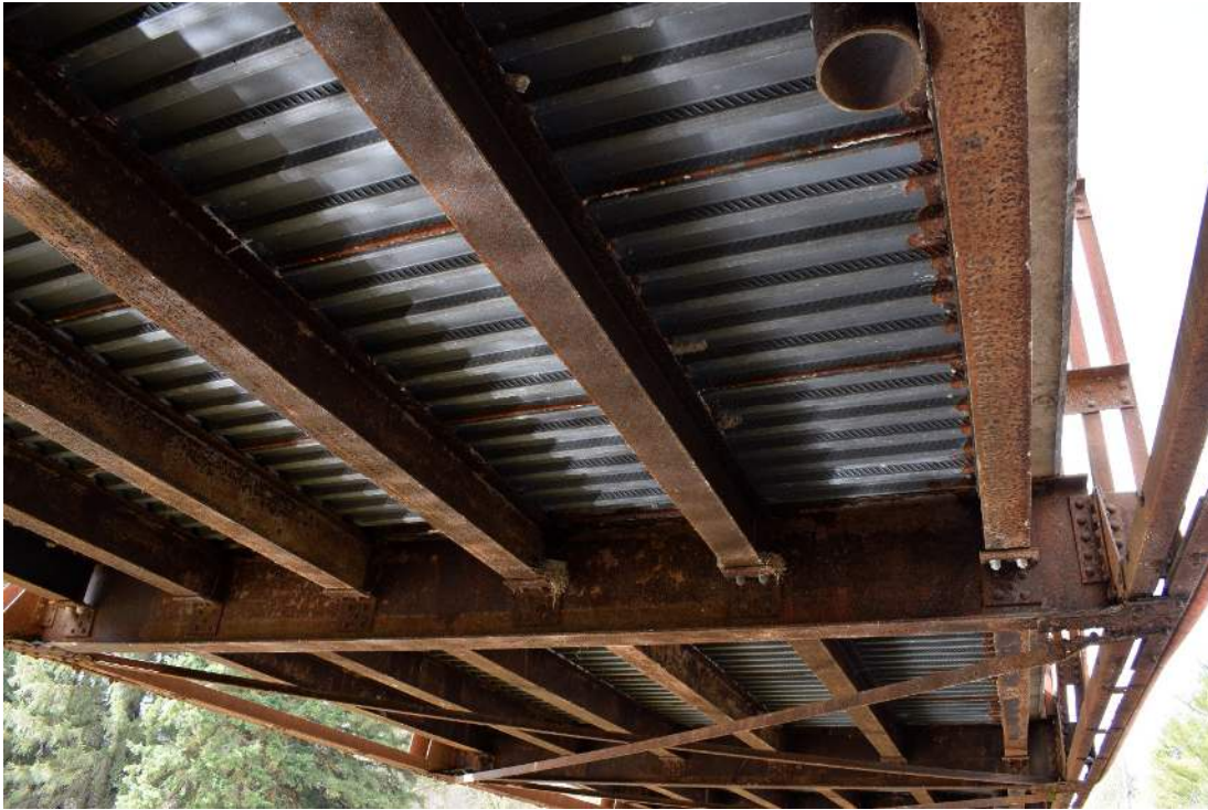
Figure 47: Underside of bridge deck, multiple signs of past repairs as evident by the use of modern bolt and not fasteners
