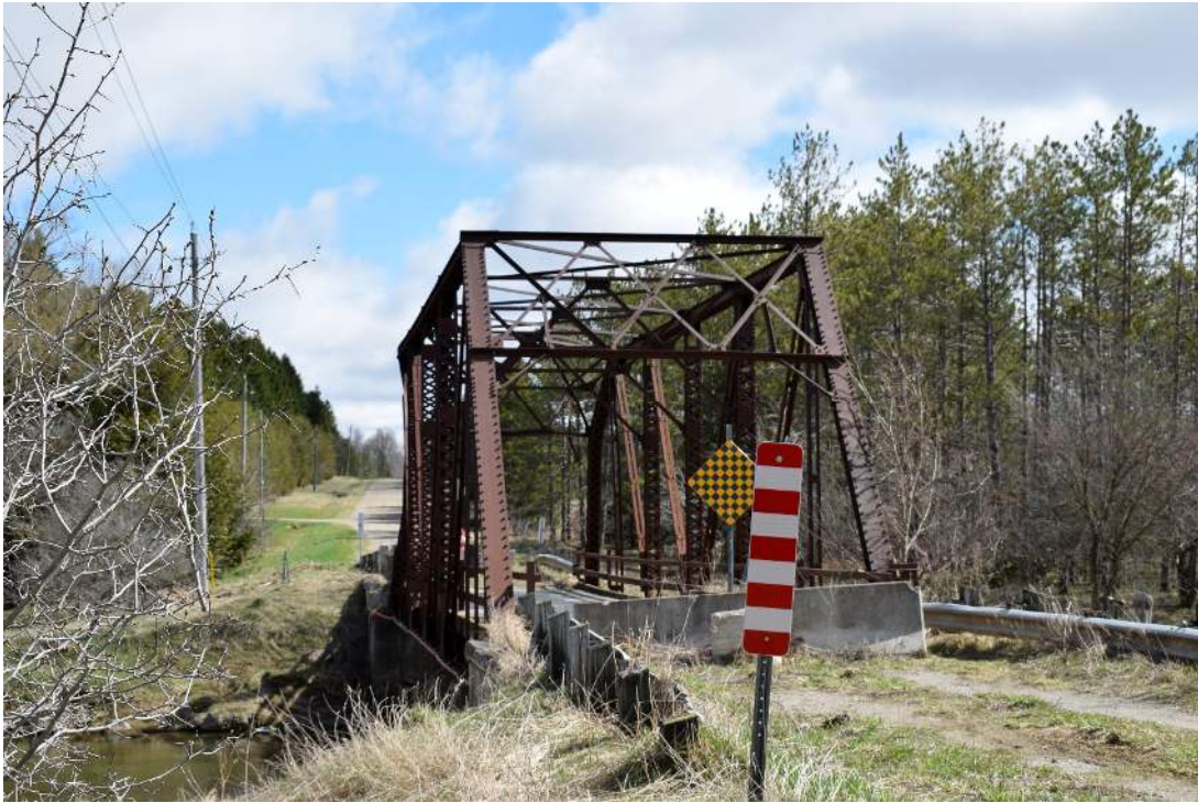
Figure 43: Eastern end of bridge which has been subject to previous restoration, with major structural components having been replaced and fastened with bolts and nuts
