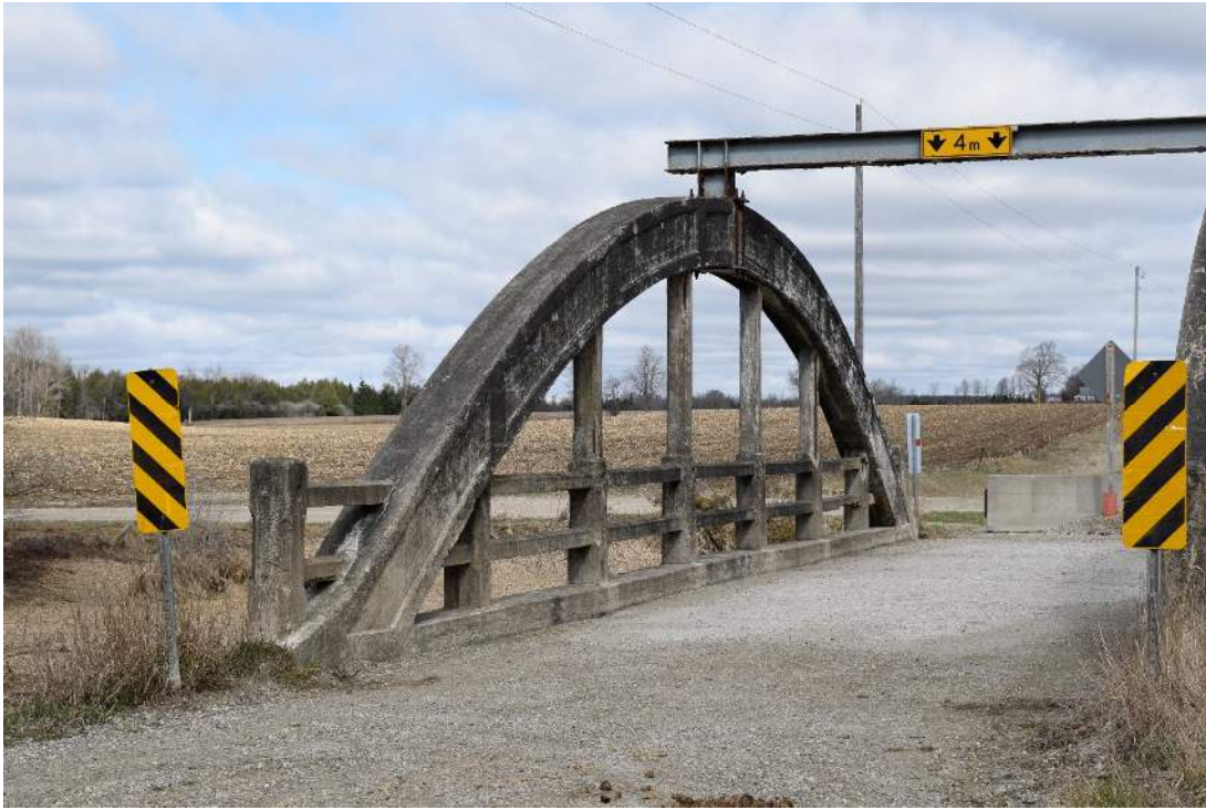
Figure 11: Western arch of Bridge 21-WG
