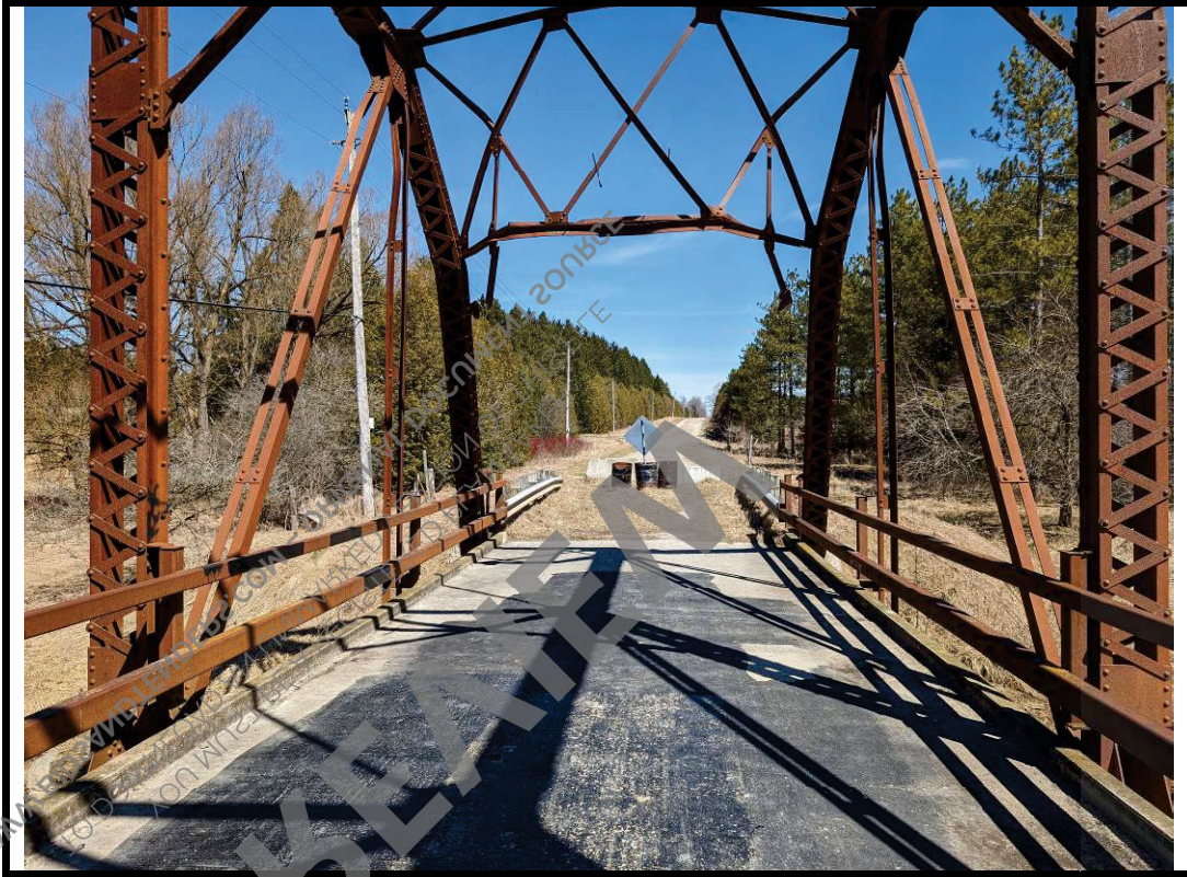
Photo 3 East approach from center of structure
