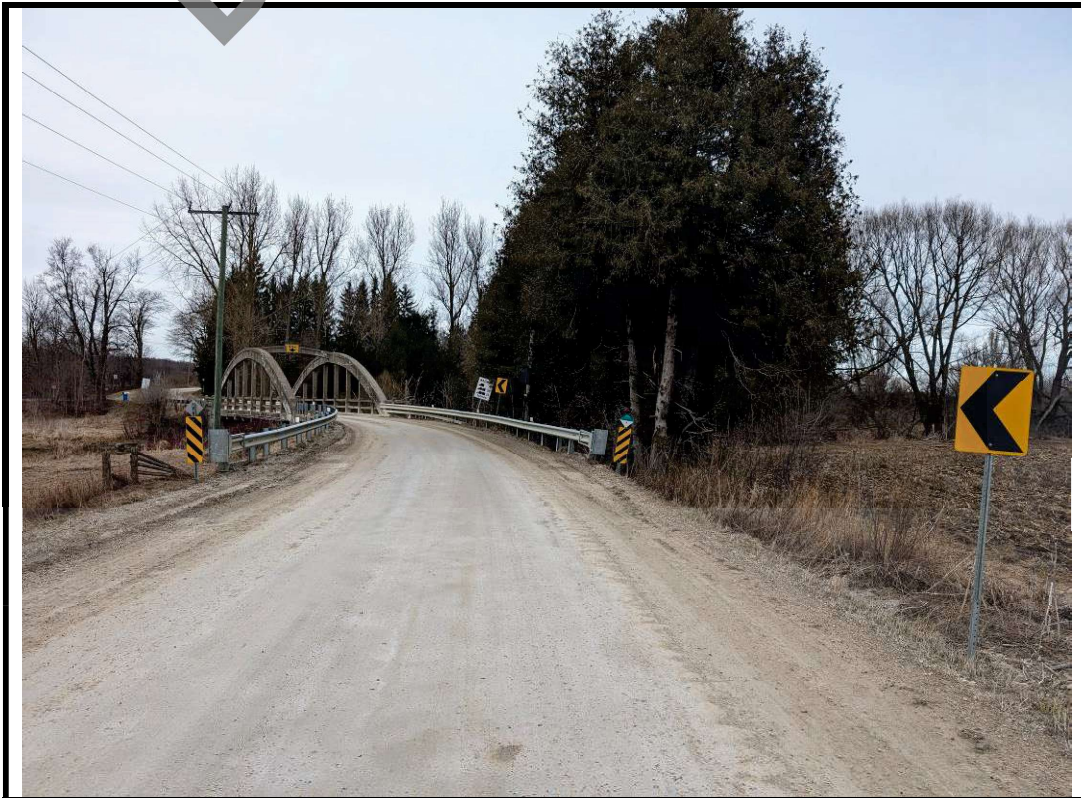
Photo 2 Structure from west approach
