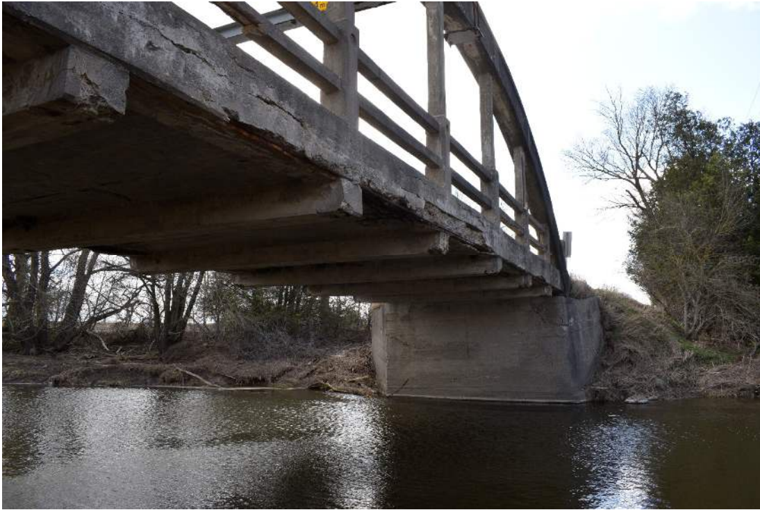
Figure 13: Underside of road deck of Bridge 21-WG and southern abutment
