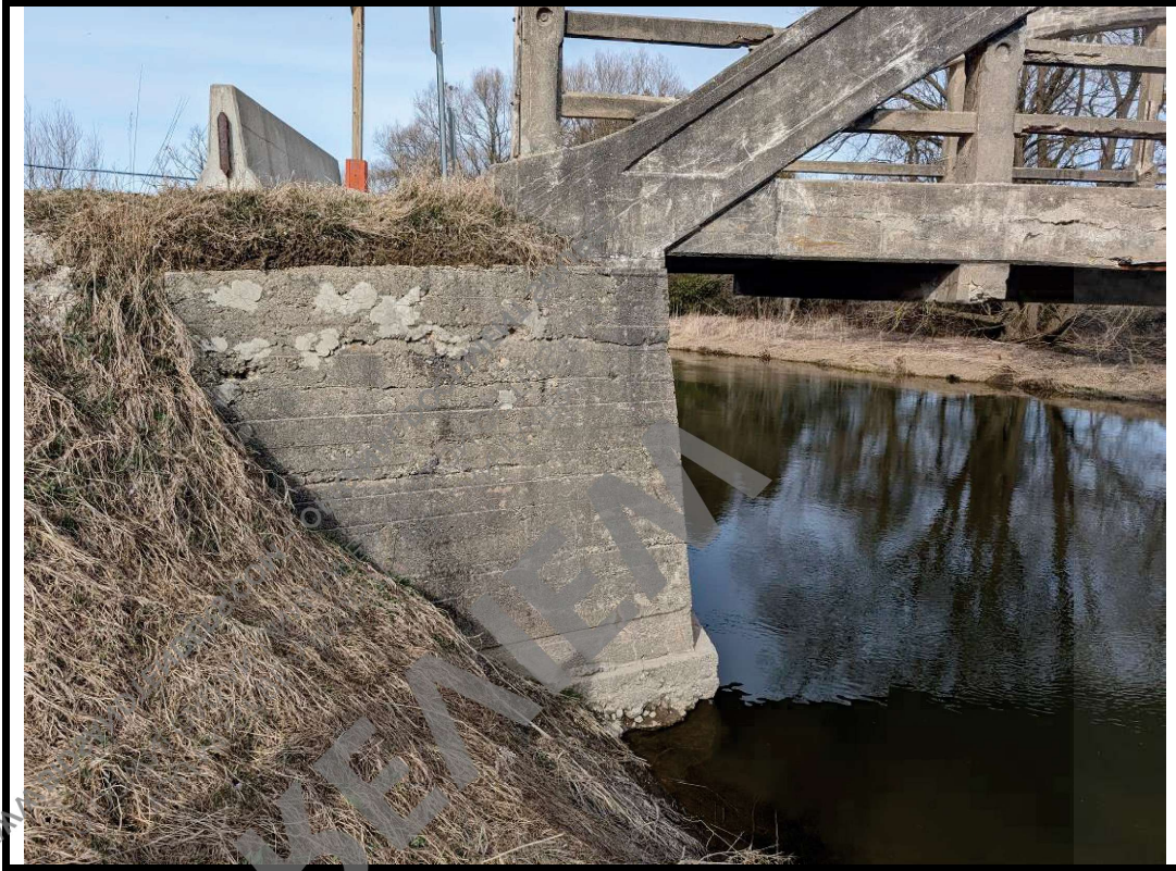
Photo 17 Wide cracks, spall and severe scaling noted on northwest wingwall
