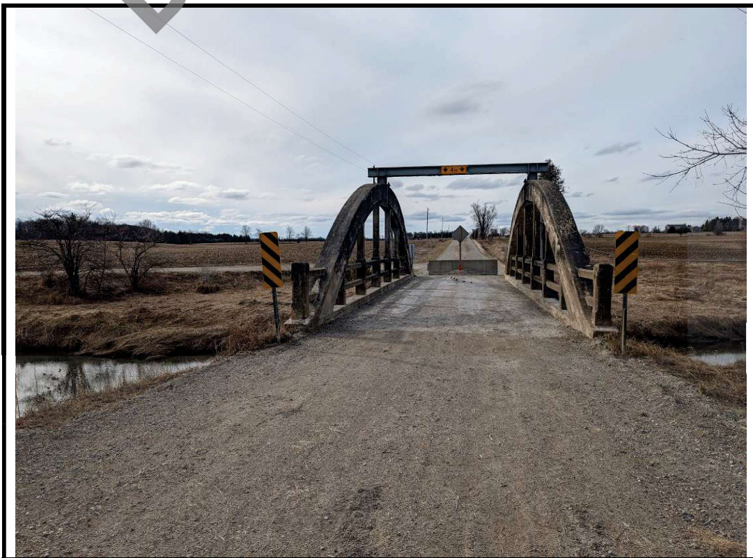
Photo 2 Structure from south approach
