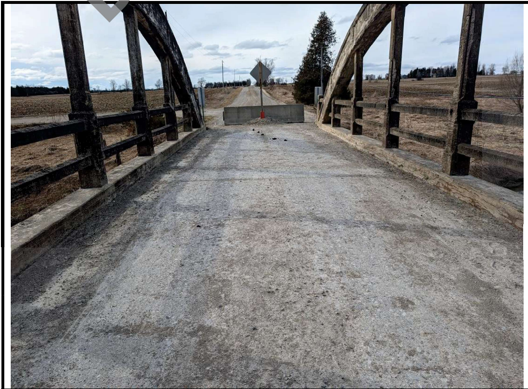
Photo 8 Moderate to severe scaling on visible portion of exposed deck top.
