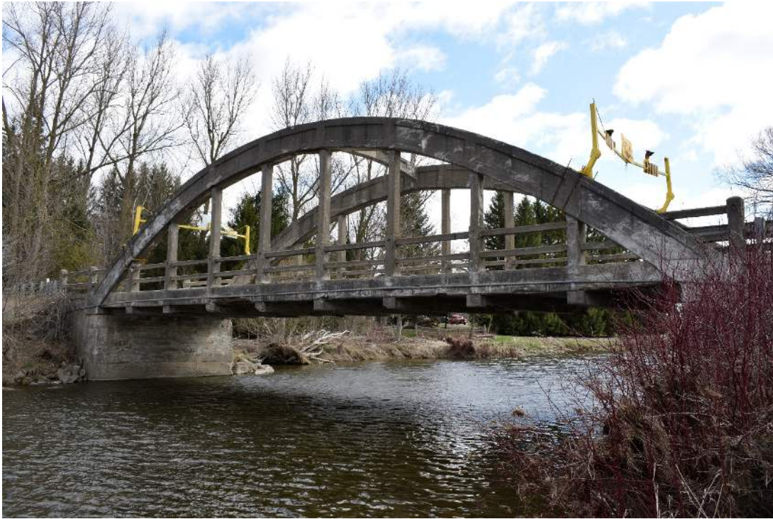
Figure 28: Southside of Bridge 29-WG
