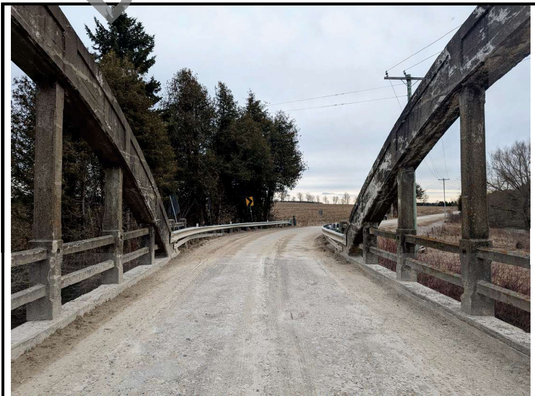
Photo 4 West approach from centre of structure
