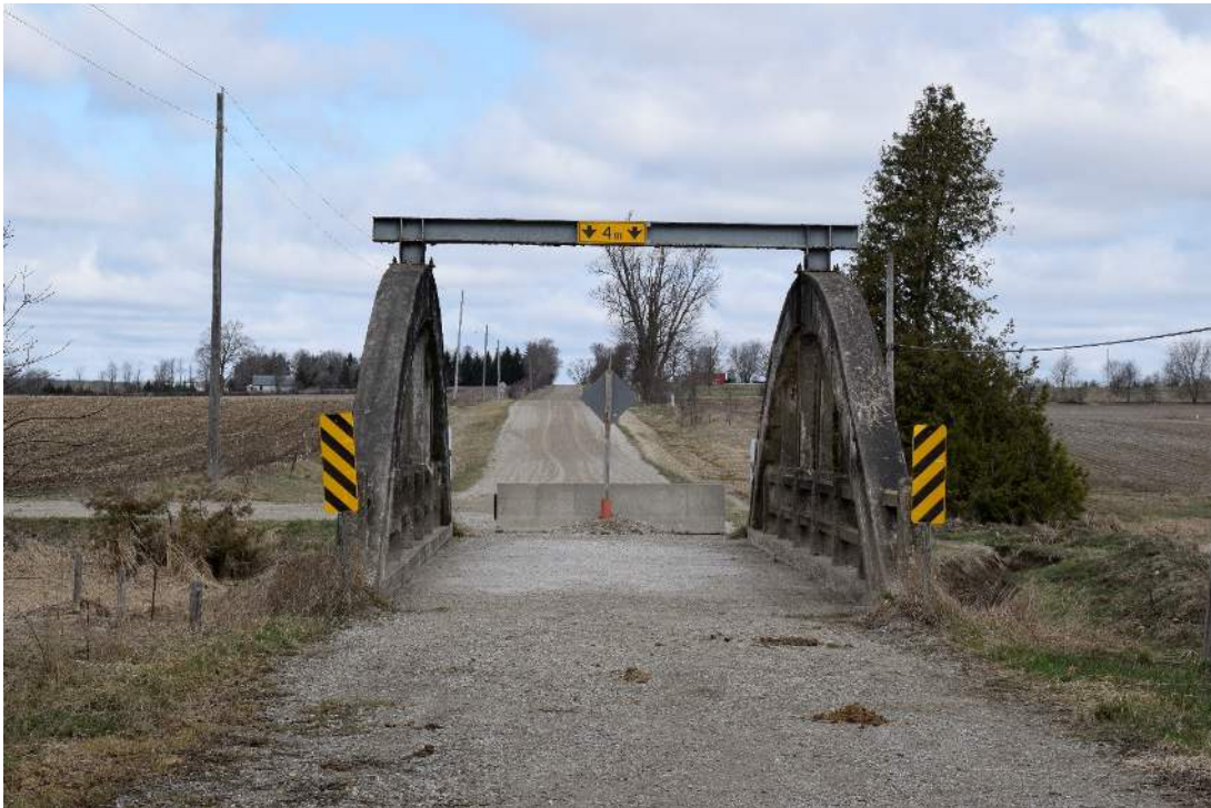
Figure 10: Southern approach to Bridge 21-WG, looking north
