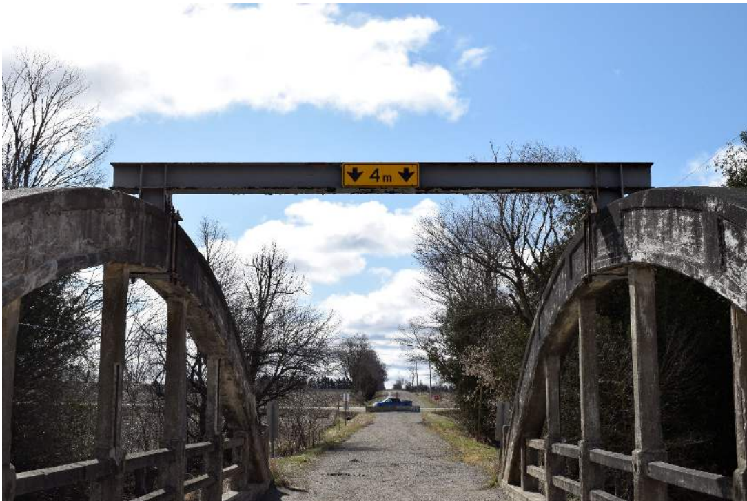
Figure 18: Retrofit steel 'I' Beam used to replace original upper cord tie
