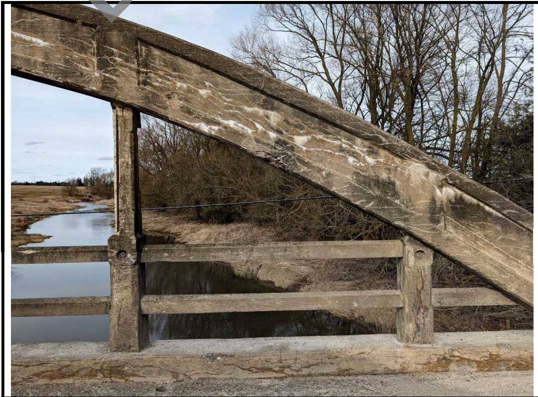
Photo 10 Wide cracks with efflorescence on east concrete arch.
