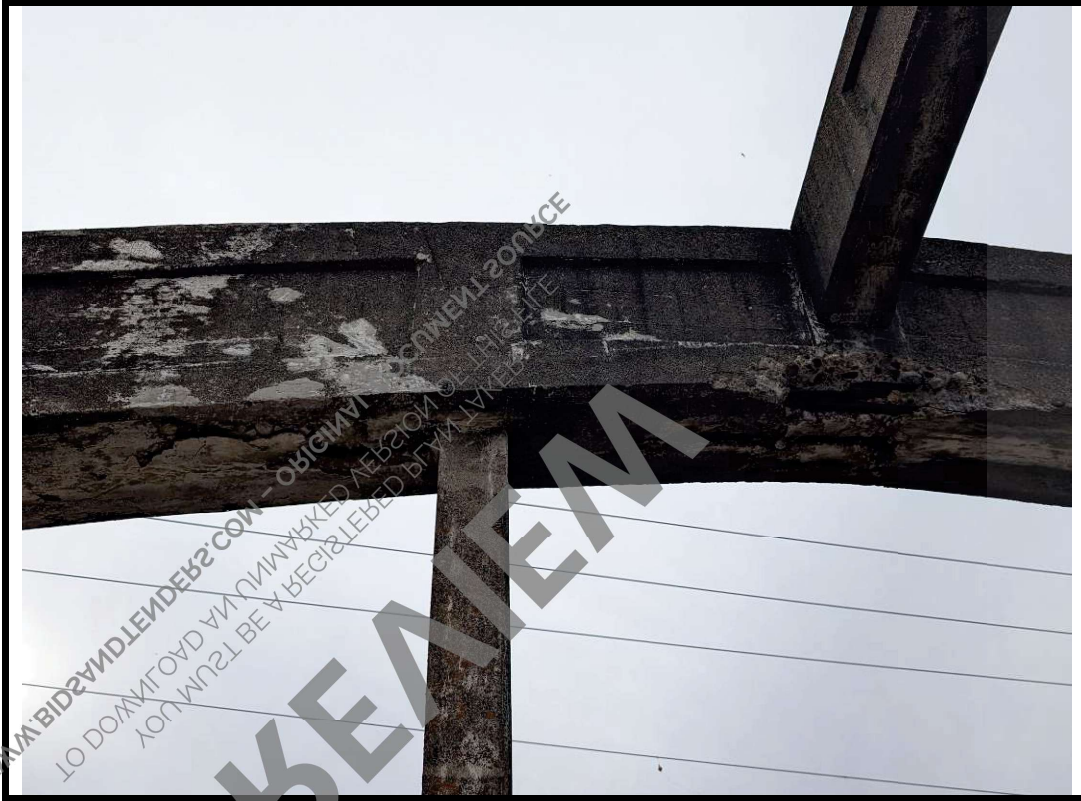
Photo 19 Small spall, scaling and narrow cracks with efflorescence stains noted on arch ribs
