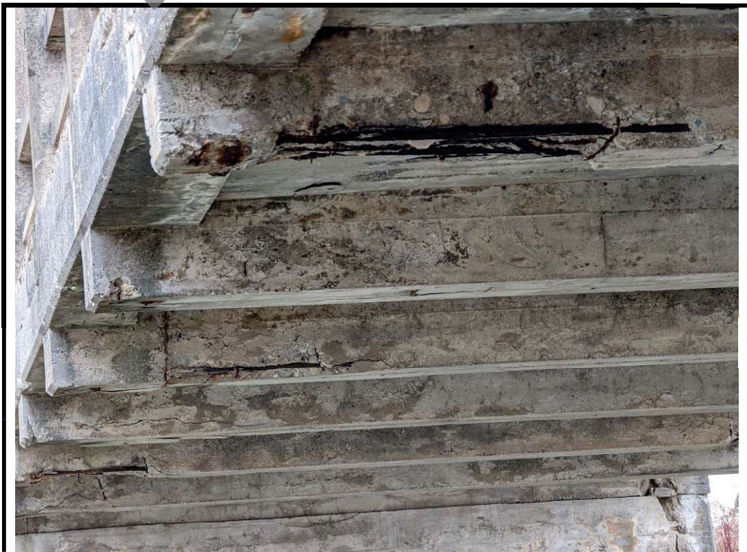
Photo 14 Typical underside of structure
