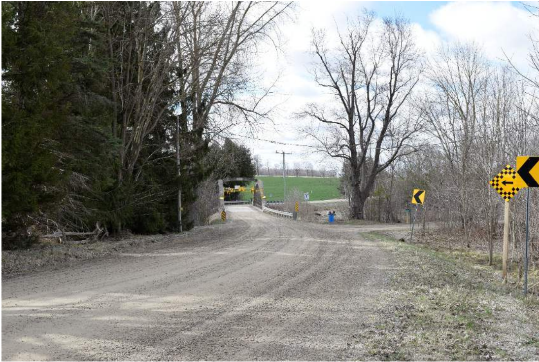
Figure 24: Western approach to Bridge 29-WG, looking west
