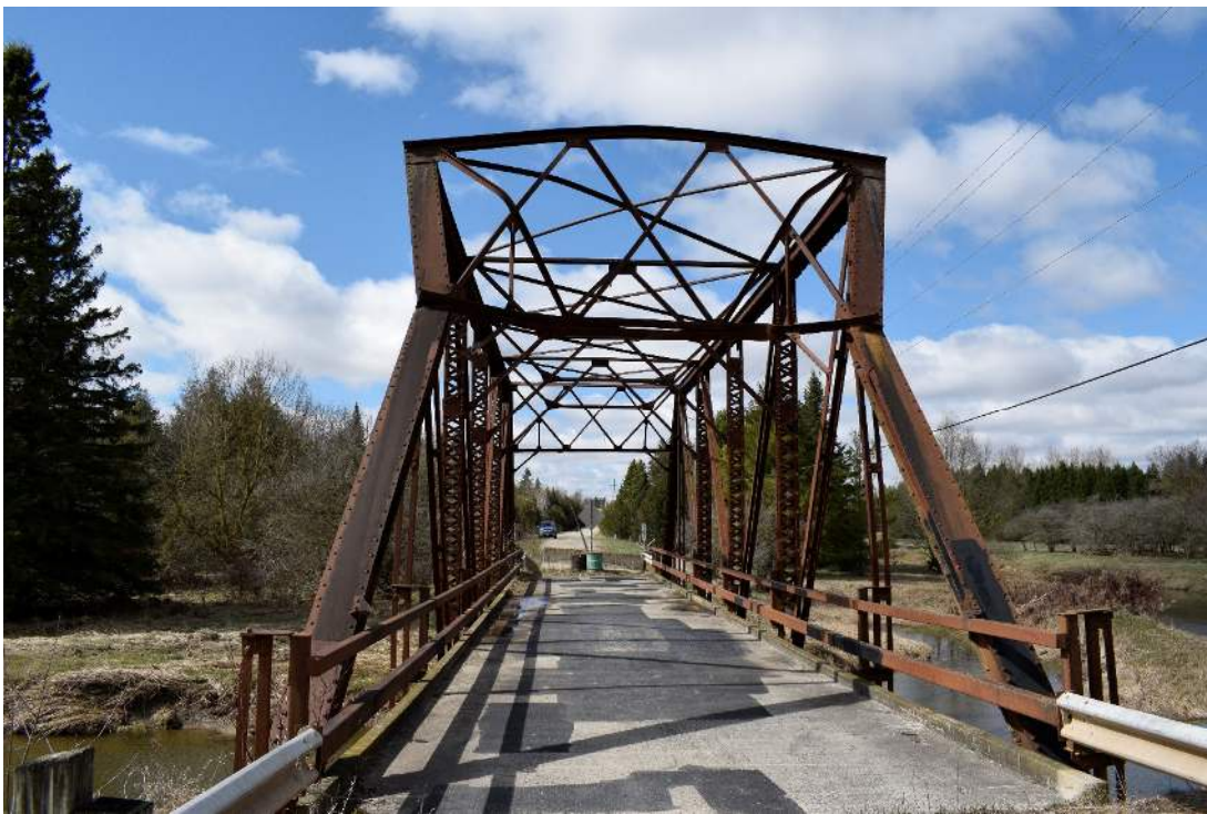
Figure 44: Western approach to bridge which exhibits deformation due to past collision with heavy equipment
