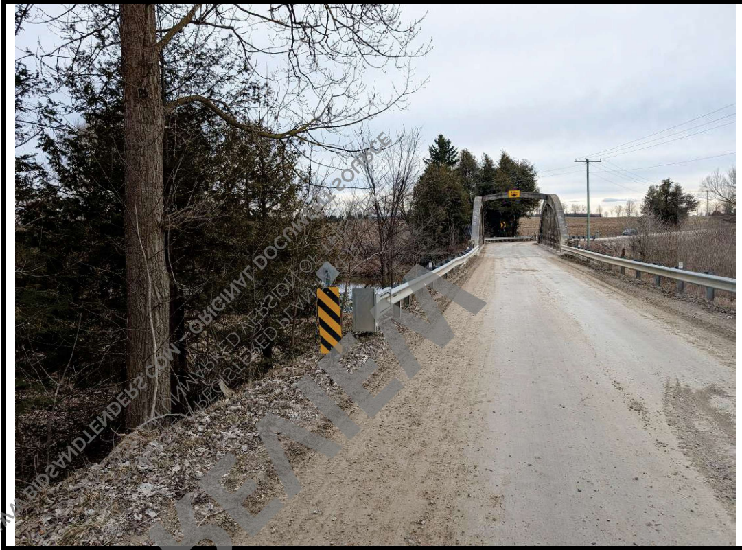
Photo 17 Typical hazard sign and end treatment at southeast corner
