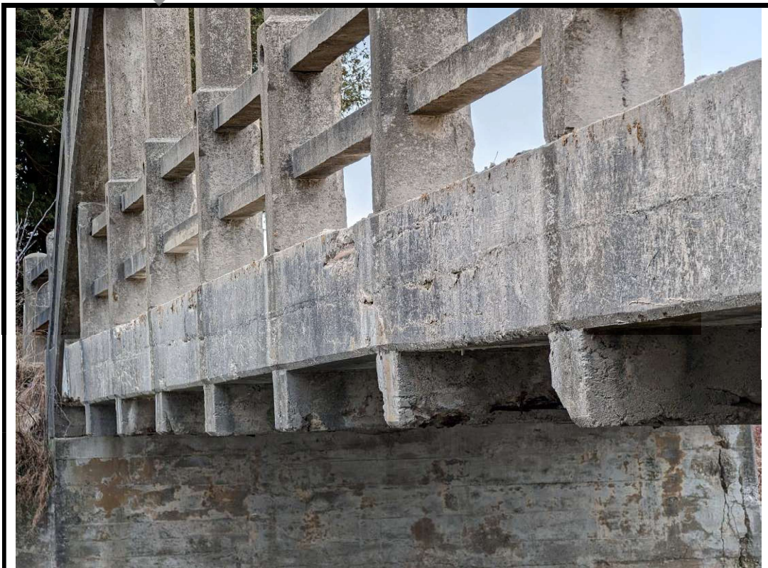
Photo 16 Cracks with stains and small spalls noted on south exterior soffit
