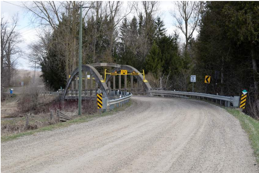
Figure 23: Eastern approach to Bridge 29-WG, looking east
