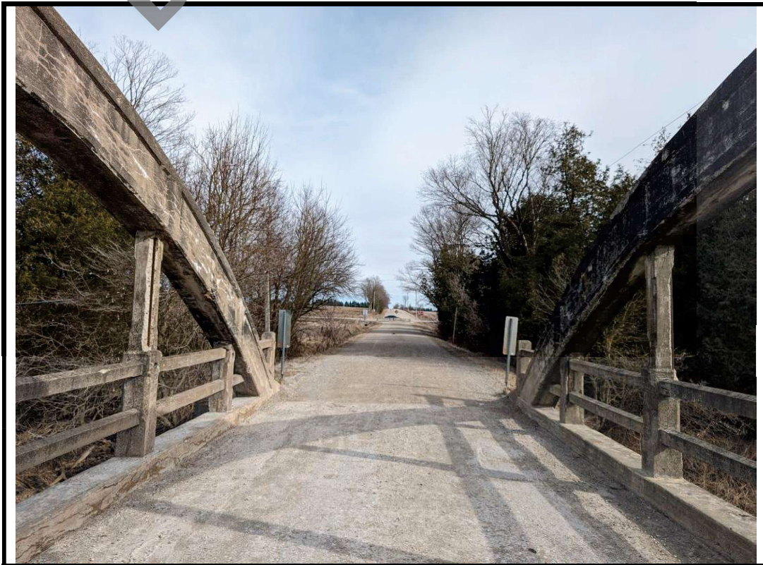
Photo 4 South approach from centre of structure
