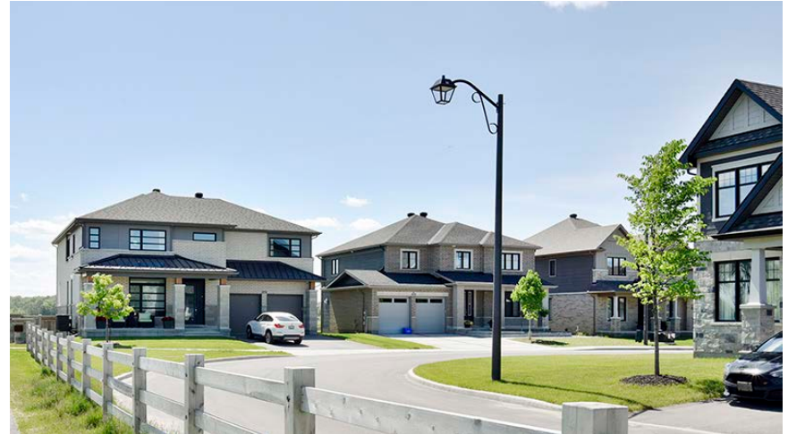
Fig.20: Traditional-style streetlights line the road, providing illumination and enhancing the streetscape (Source: GSP Group Inc.)
