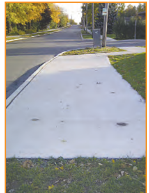
Long view of accessible bus stop pad.
