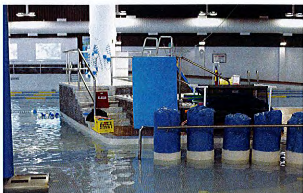
Photo 25: Pool Basin - Signage
