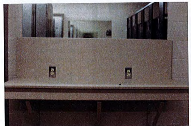
Photo 12: Female Change Room - Electrical Outlets
