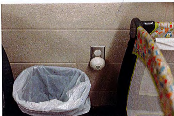
Photo 11: Female Change Room - Electrical Outlets
