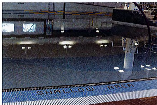
Photo 24: Pool Basin - Signage
