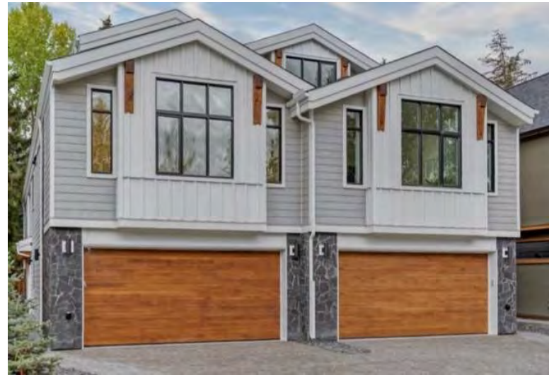
Example of Themed Exterior Finishing (Source: Strata Development Corp.)
