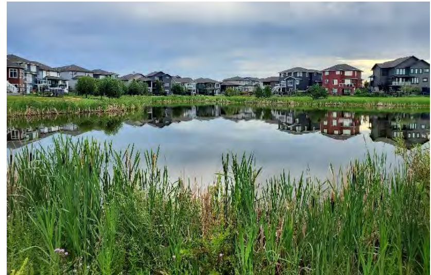
Naturalized Stormwater Management Facility (Source: Strata Development Corp)
