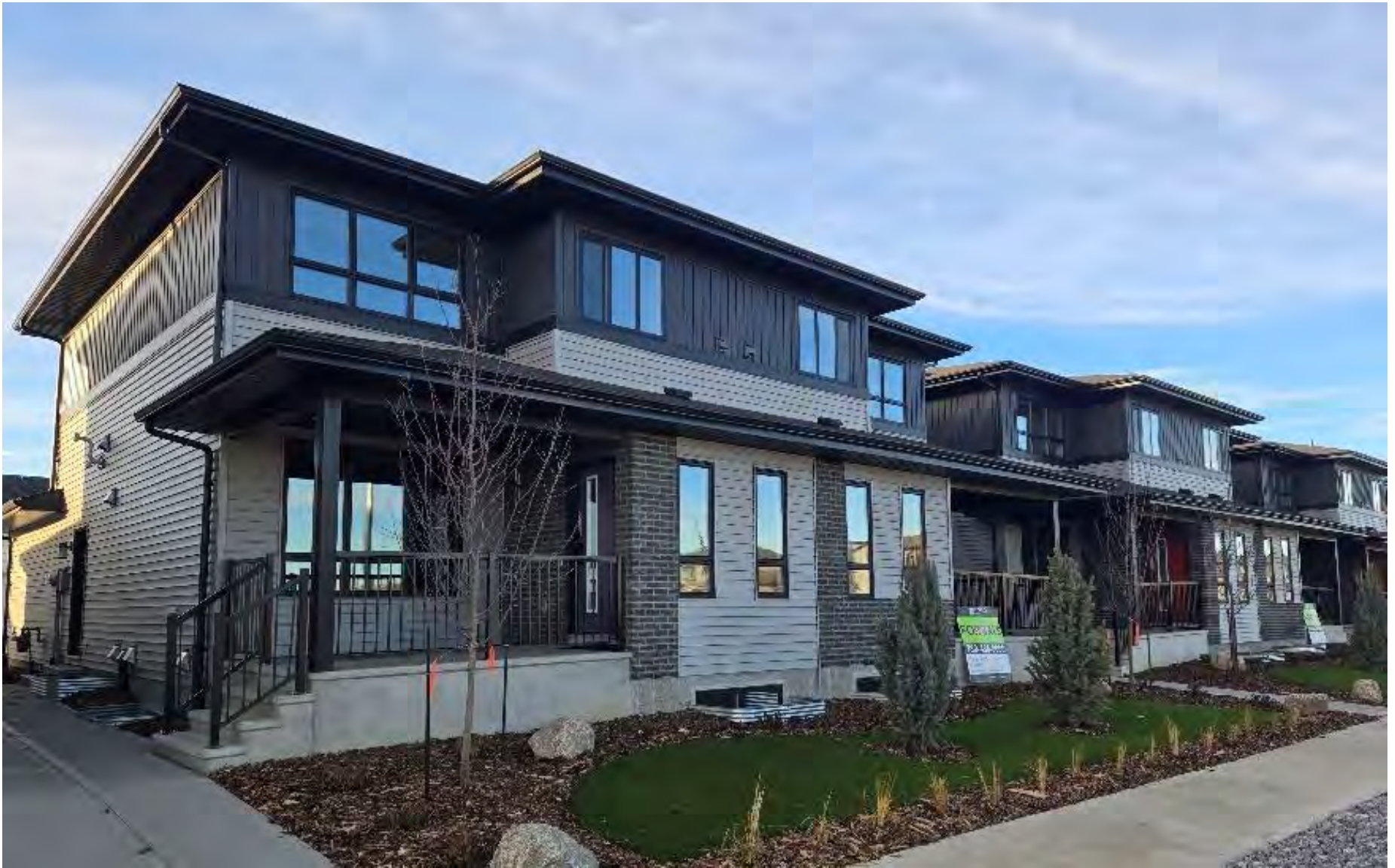
High Density Shallow Lot Residential, Fort Saskatchewan (Source: Strata Development Corp)
