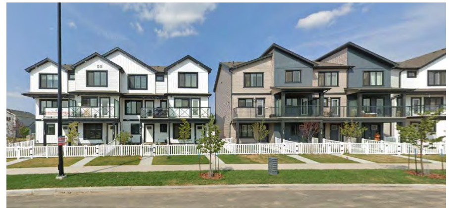
Street Oriented Narrow Lot (14' Wide) Townhouses (Source: Google Maps)
