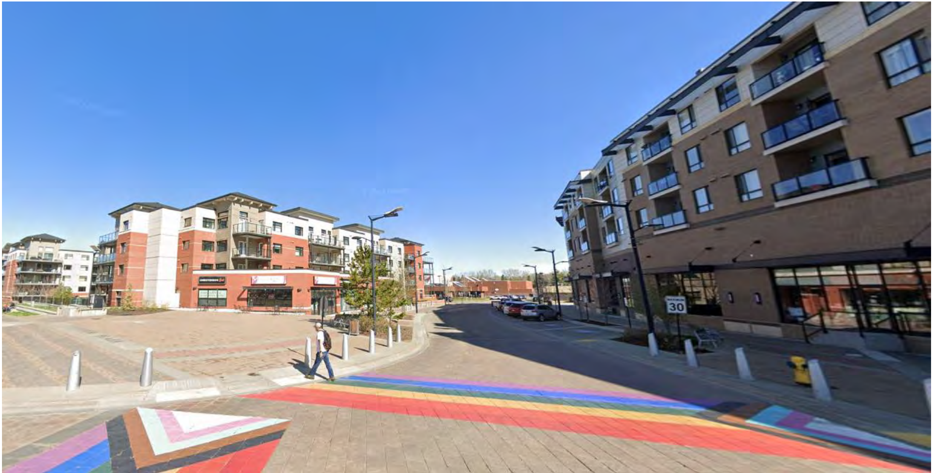
Savona Mixed-Use and Plaza – Sherwood Park, AB (Source: Google Earth)
