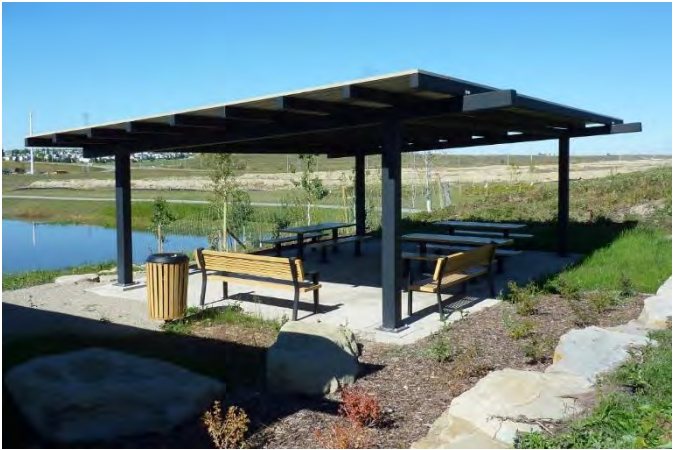
Figure 2 – Example of a shade shelter
