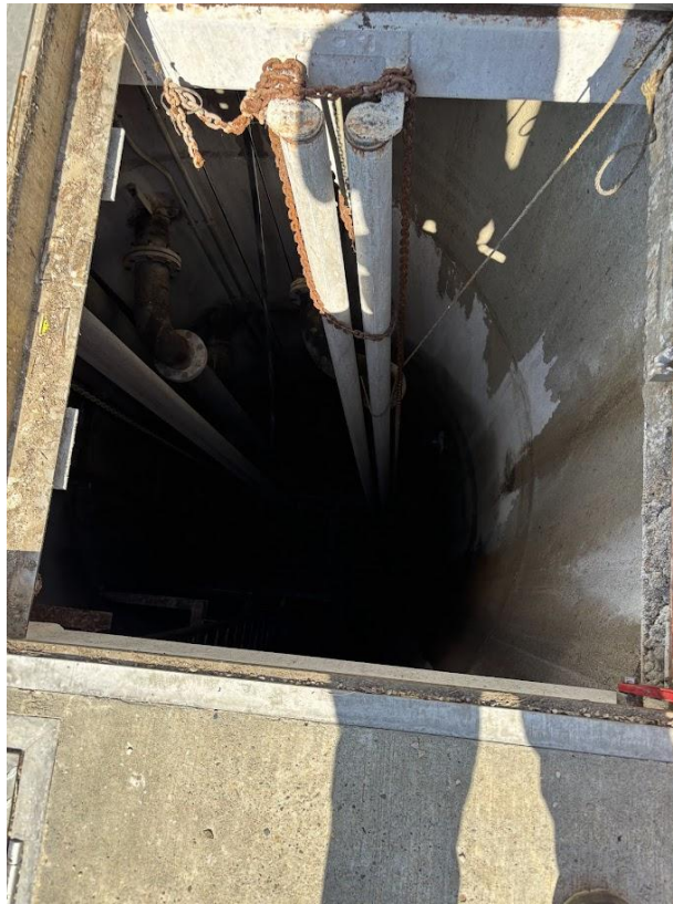
View of the wet well entrance from ground level
