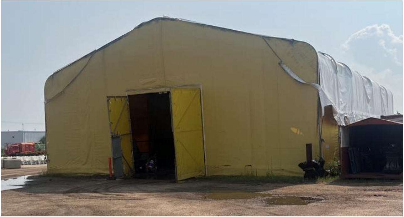
Existing Parks Quonset – Exterior
