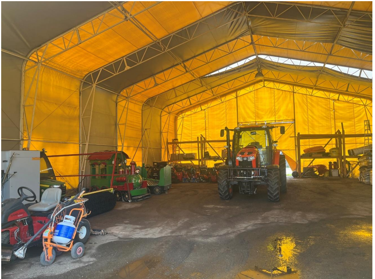
Existing Parks Quonset - Interior
