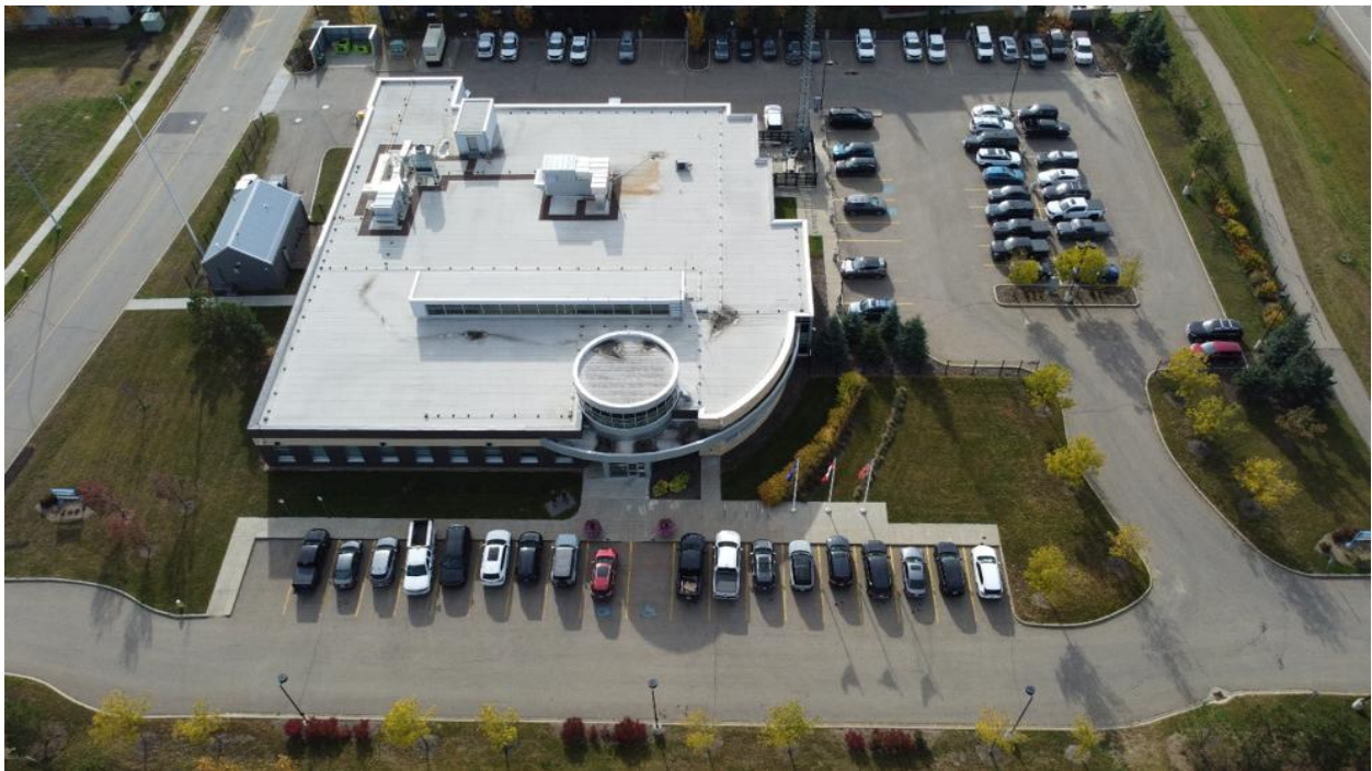
The above photo shows the parking congestion at the Protective Services Building.
