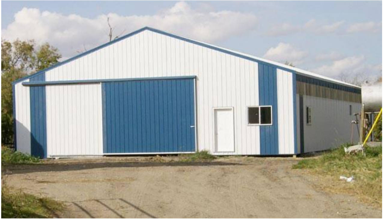
Example of Hard-walled Quonset - Exterior
