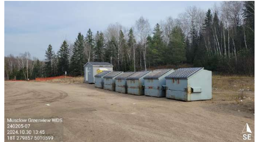
Photo 14: Attendant's building and recycling depot – October 30, 2024
