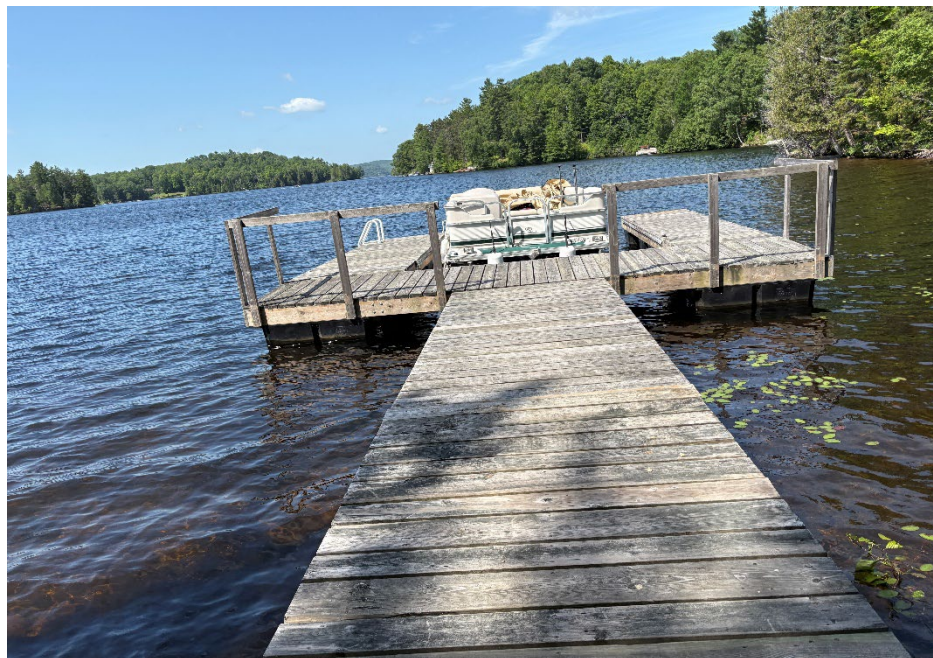
Photo 3 Existing dock structure, July 2026.
