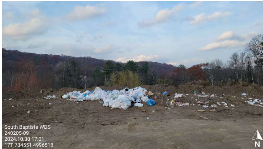
Photo 29: Active landfill cell – October 30, 2024
