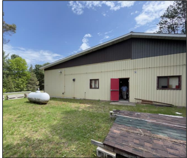
Rear of fire Station
