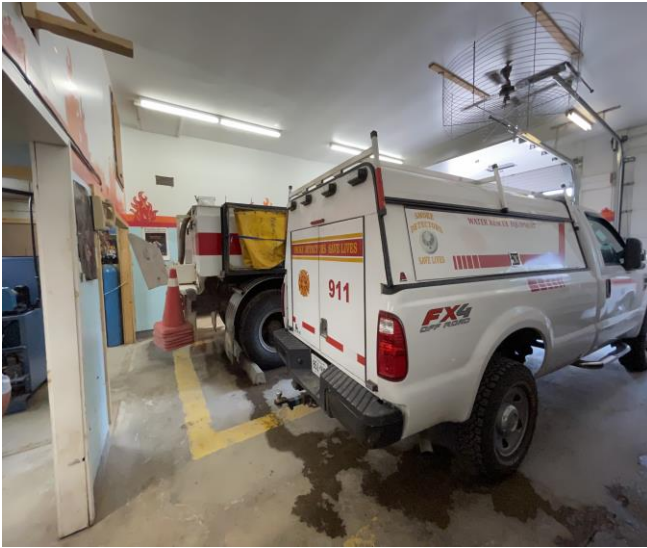
Apparatus Bay & Air Filling System
