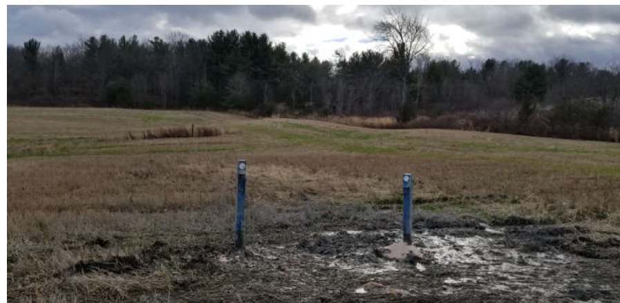
12. Newly installed MW105 (Left) and MW106 (Right) November-2022
