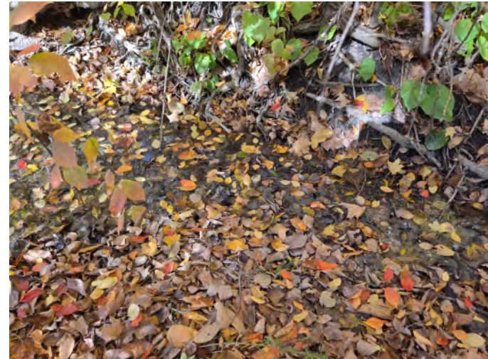
10. Hickenbottom® Drain Outlet. (October 2024)
