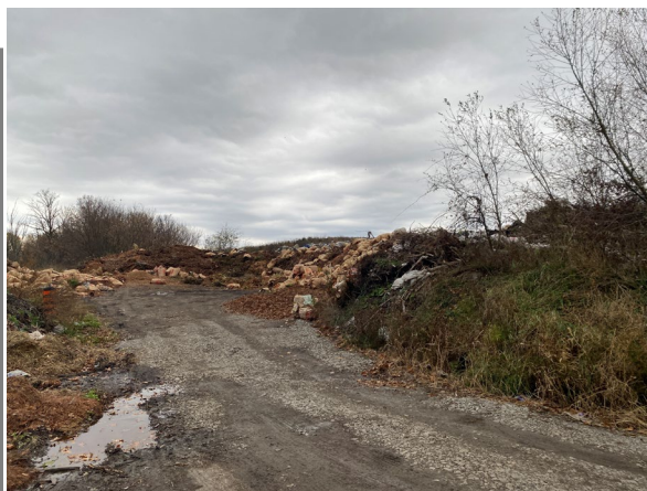
Photo 4: Berm of leaf and yard waste pushed up against northeast side of landfill facing south. Pool of leachate visible at bottom left of photo.
