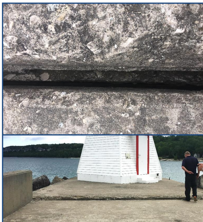
Figure 7-1: Separation of Concrete Lighthouse Base Slab from Concrete Wharf
