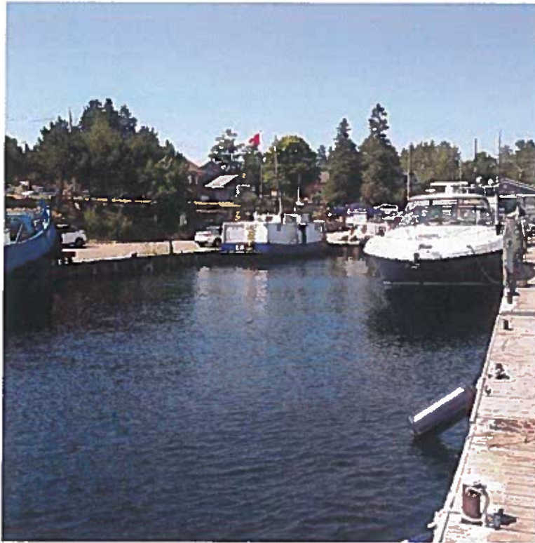
Figure 5: Steel Dock 3-4 and South Wharf, Looking West
