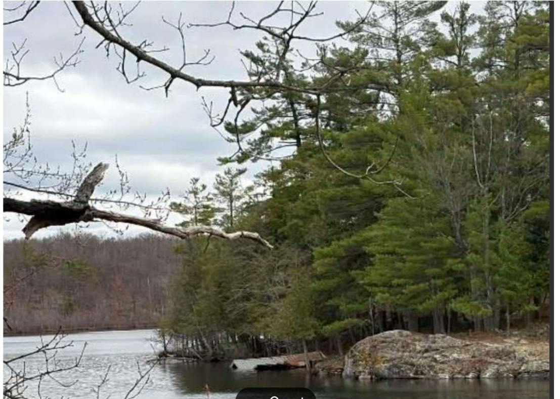
Existing Picture – Spring 2026 (Boathouse collapsed into water)
