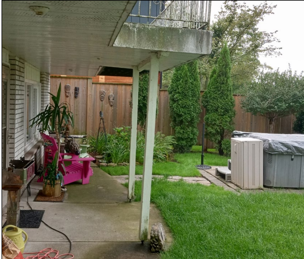
Figure 4: Underside of Deck and Supporting Posts
