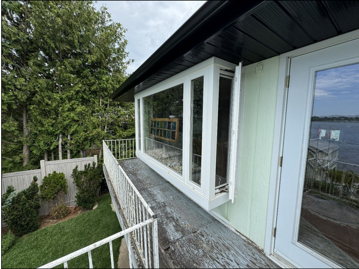
Figure 8 – Existing Deck in Front of Bay Window (Applicant Photo)
