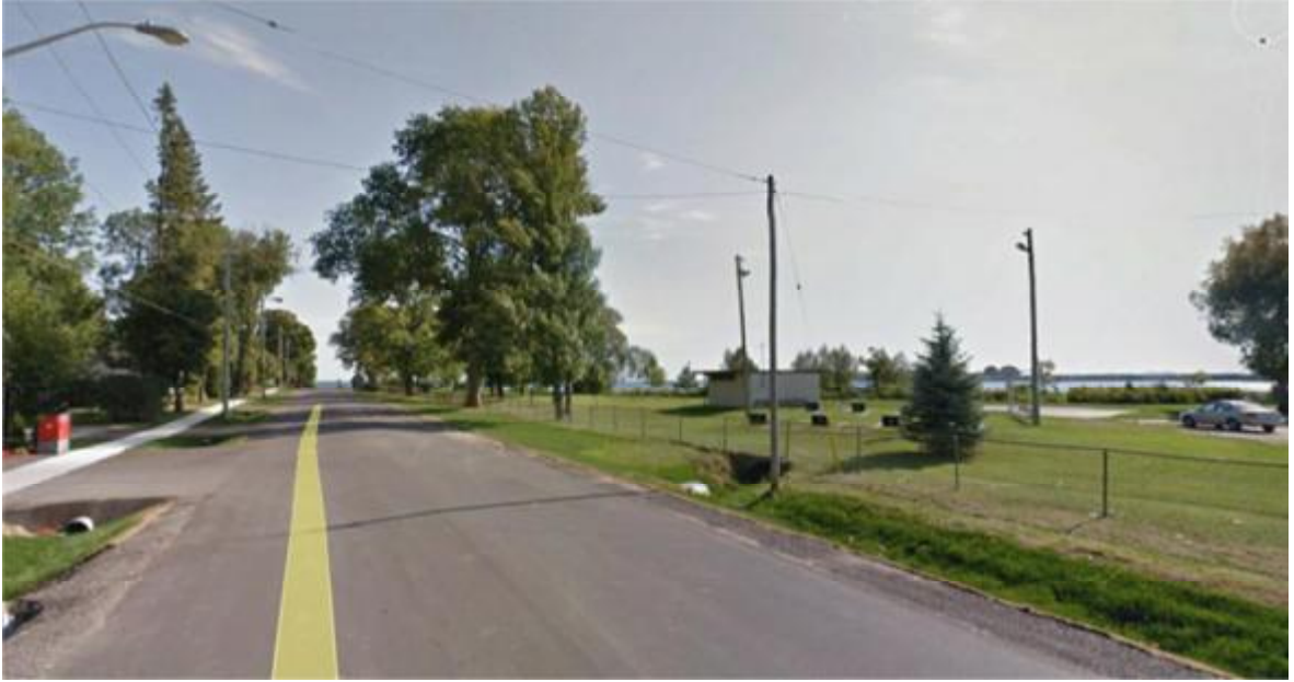
Outfall from West St. S. into Kitchener Park
