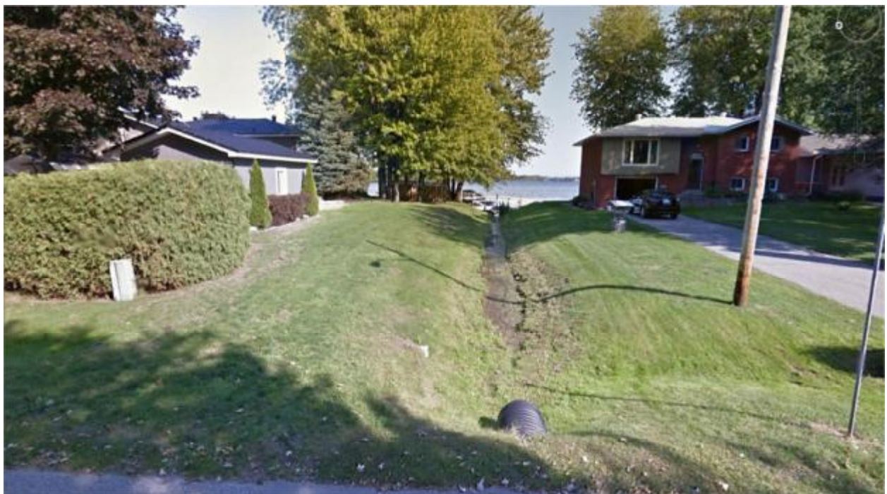
Outfall No. 75 on east side of Collins Dr.
