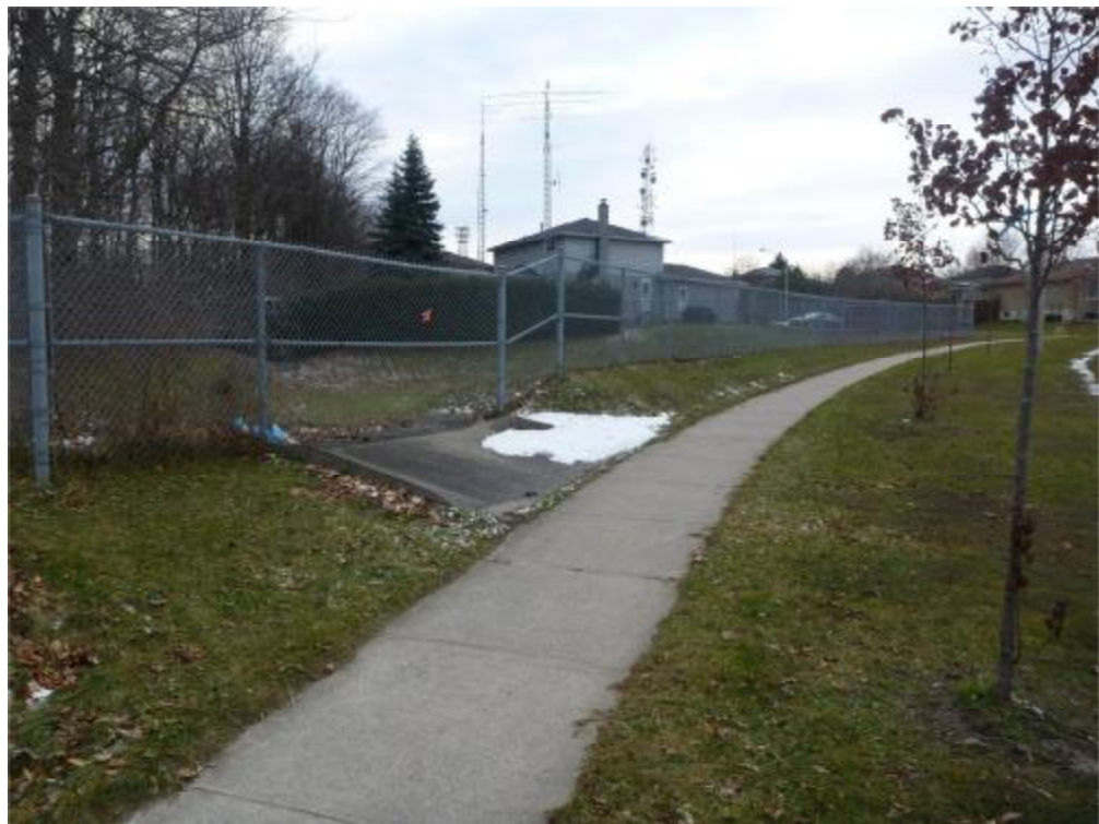
F7 - Overflow to Woodside Drive
