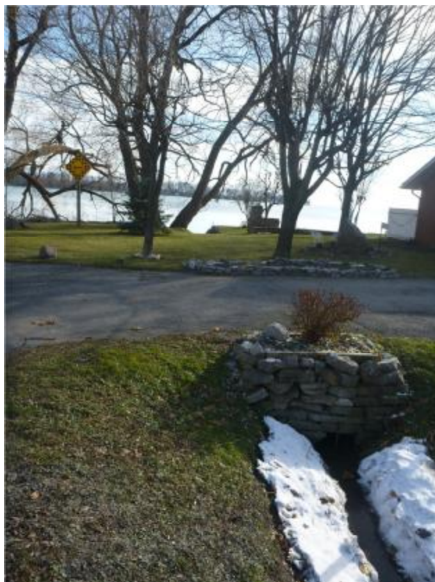
Outfall through front yard on Gill St.
