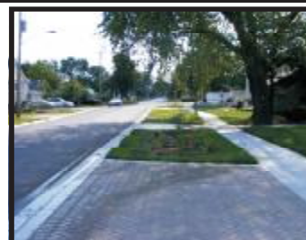
Planted Garden Bioretention
