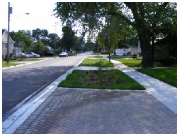
Planted Garden Bioretention
