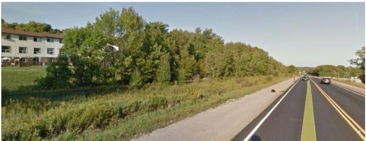
Ditch on N. side of Highway 12, south of Walker Ave.
