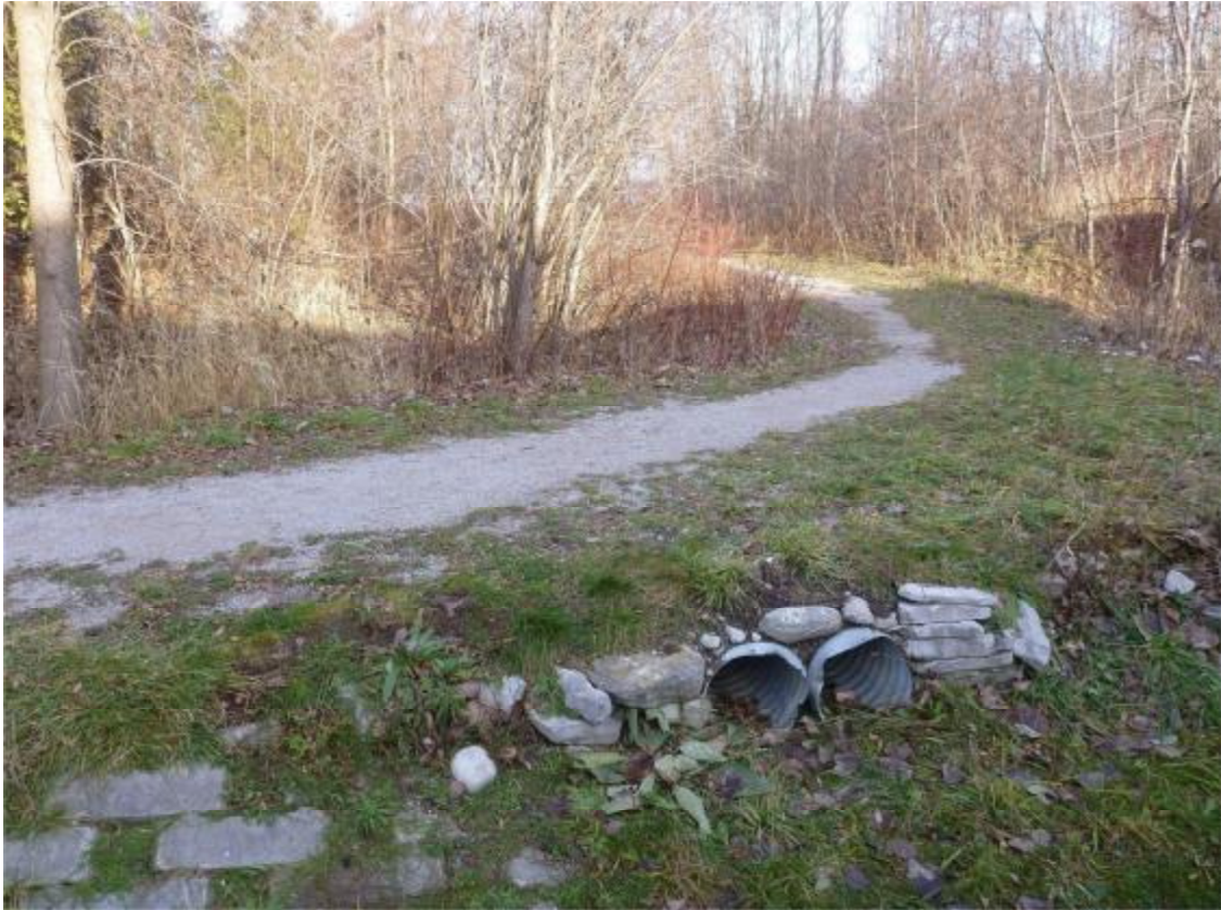
Culverts to outfall channel No. 43 adjacent to path
