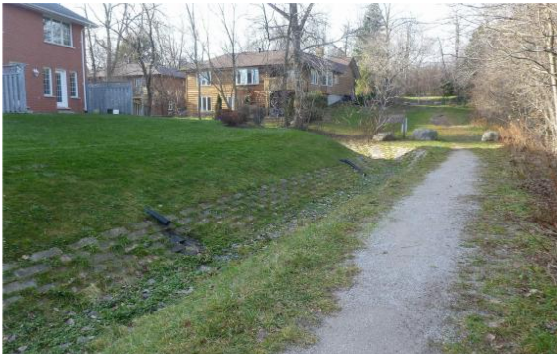
Upstream terrafix-block lined ditch draining to Outfall No. 43
