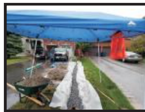
Soakaway Pit/ French Drain Retrofit - During and After (L to R)
