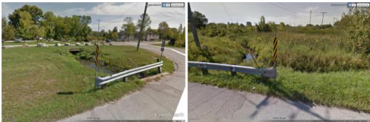
Channel to Outfall No. 31 at Cedar Island Road: Left = downstream, Right = upstream
