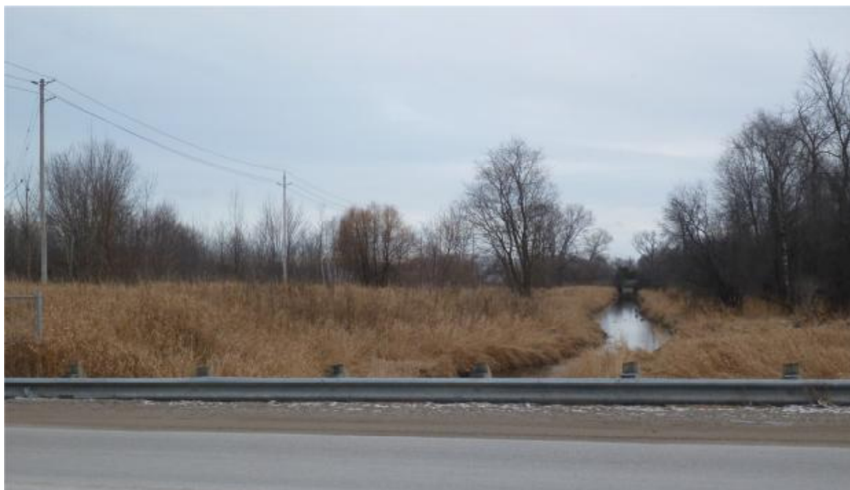
Ben's Ditch looking downstream from James St. toward Highway 12
