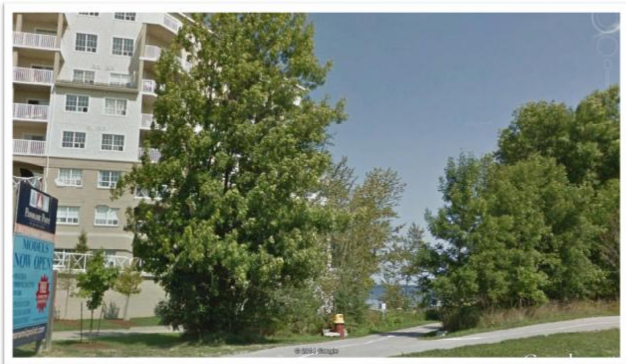
Outfall No. 46 adjacent to path north of Atherley Rd.
