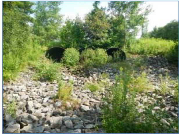
Silver Creek Stormwater Outlet Protected by RipRap.
