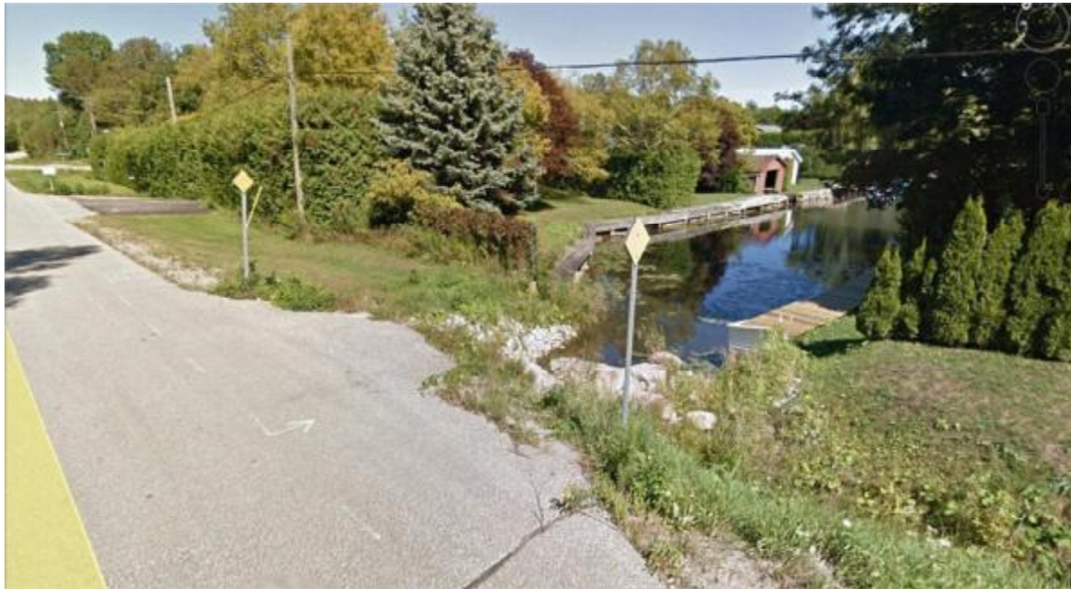
Outfall No. 1 on downstream (east) side of Drinkwater Dr.
