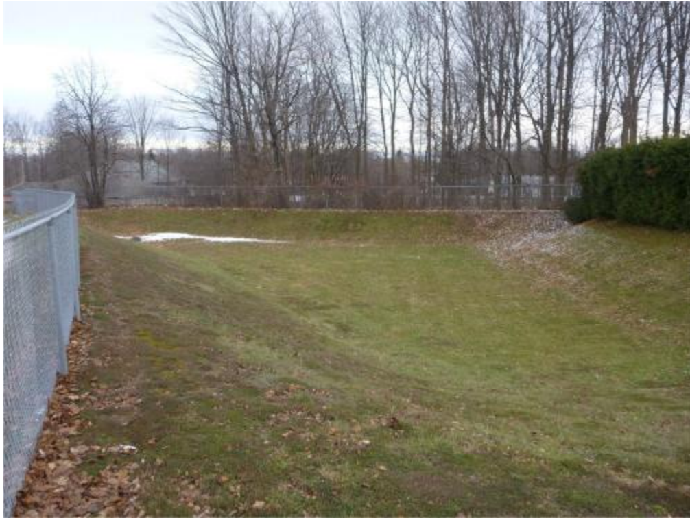
Existing Dry Pond F7
