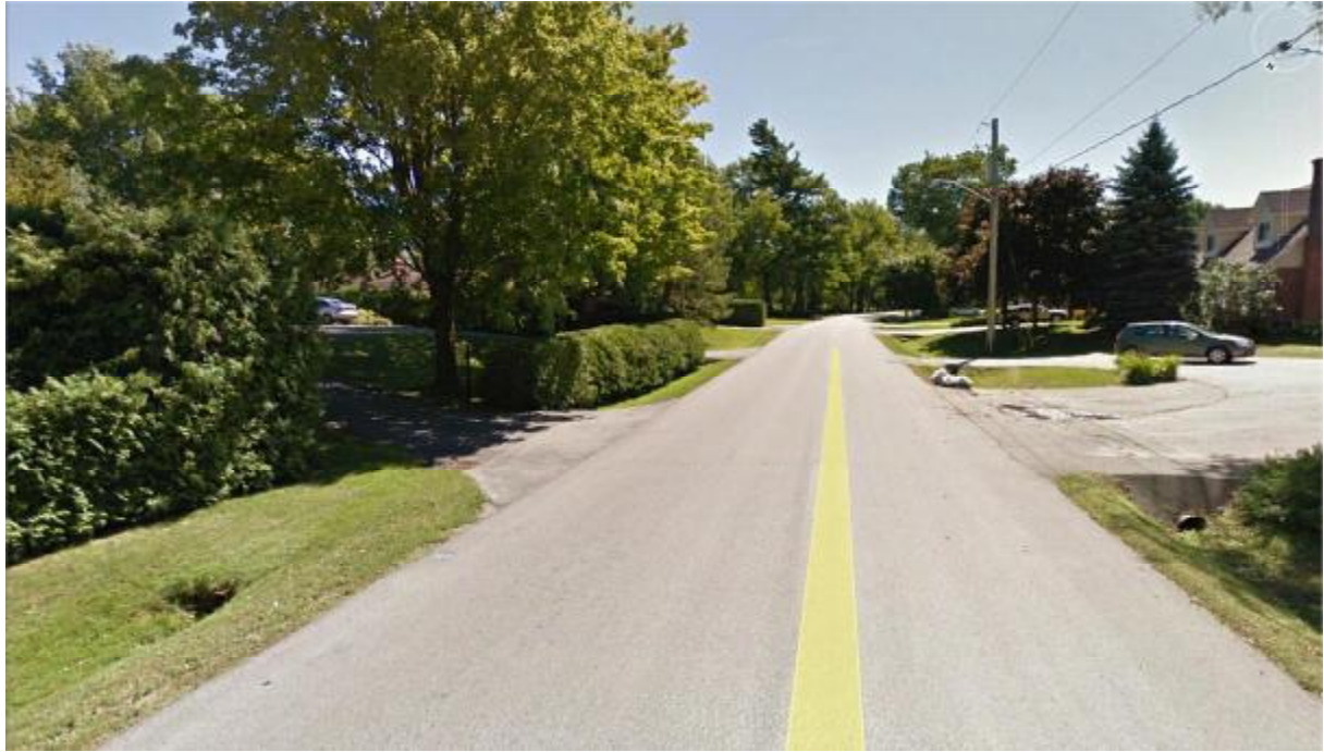
Roadside ditch drainage on Maple St. to Outfall No. 6
