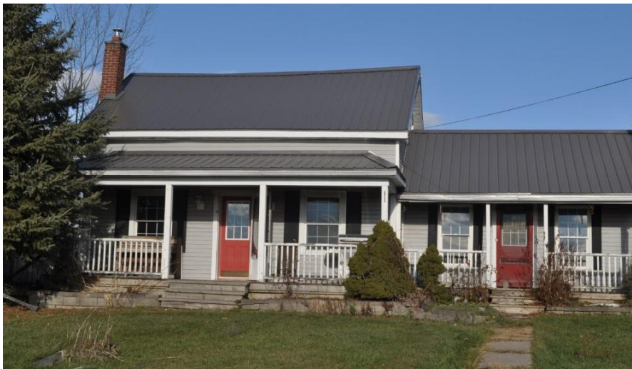
Figure 15. The Stone Mills Fire Department's training house.
