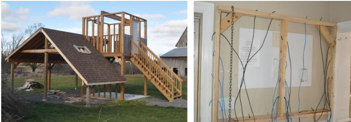
Figure 17. The Stone Mills Fire Department's training props.
