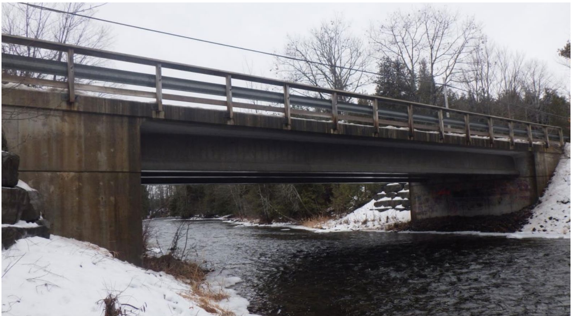
Figure 3-3: Example of Good Condition Bridge or Culvert – Adair Bridge
