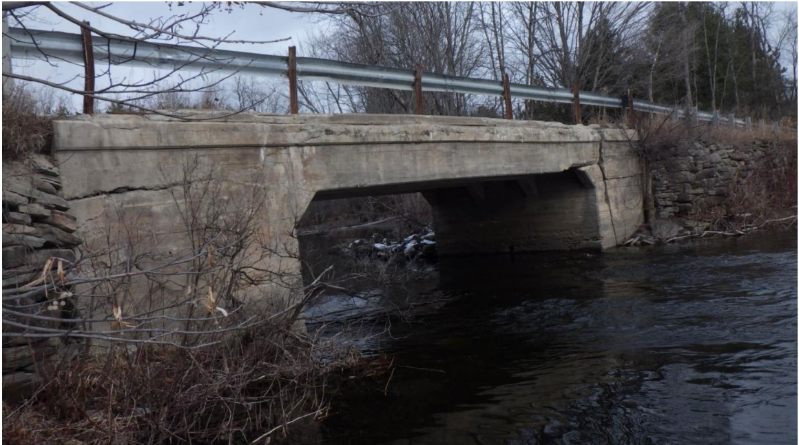
Figure 3-2: Example of Fair Condition Bridge or Culvert – Kirk's Bridge
