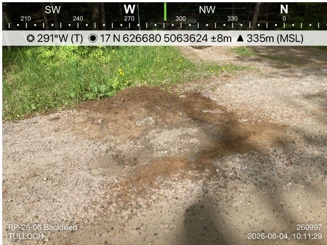
Photo 22: RP-26-06 Backfilled and Completed
