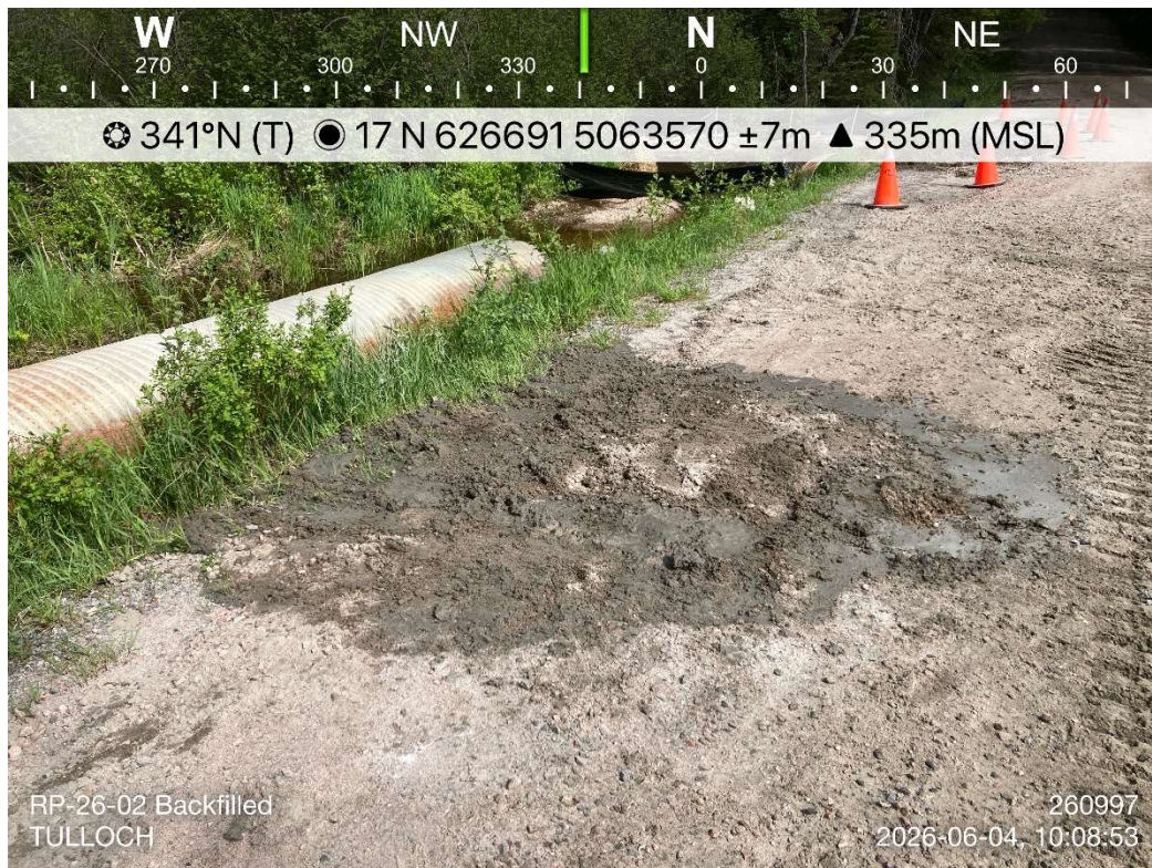
Photo 14: RP-26-02 Backfilled and Completed
