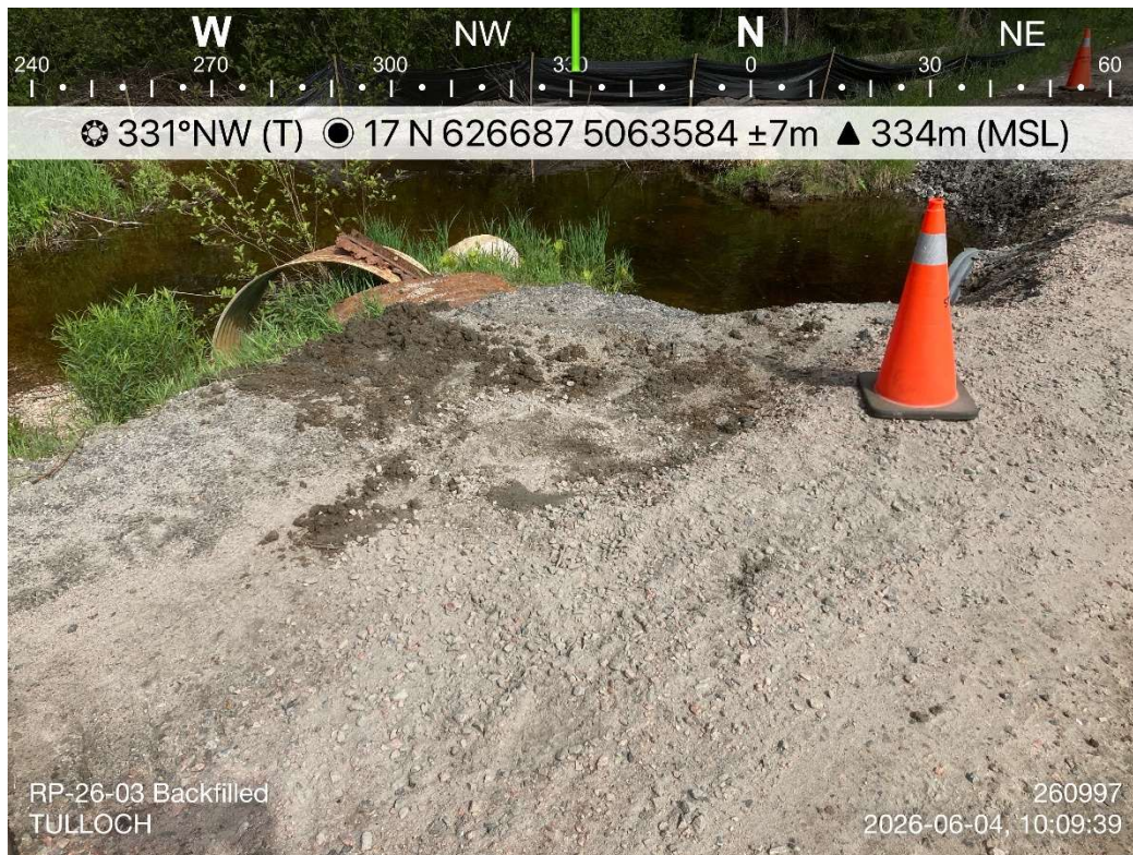
Photo 16: RP-26-03 Backfilled and Completed
