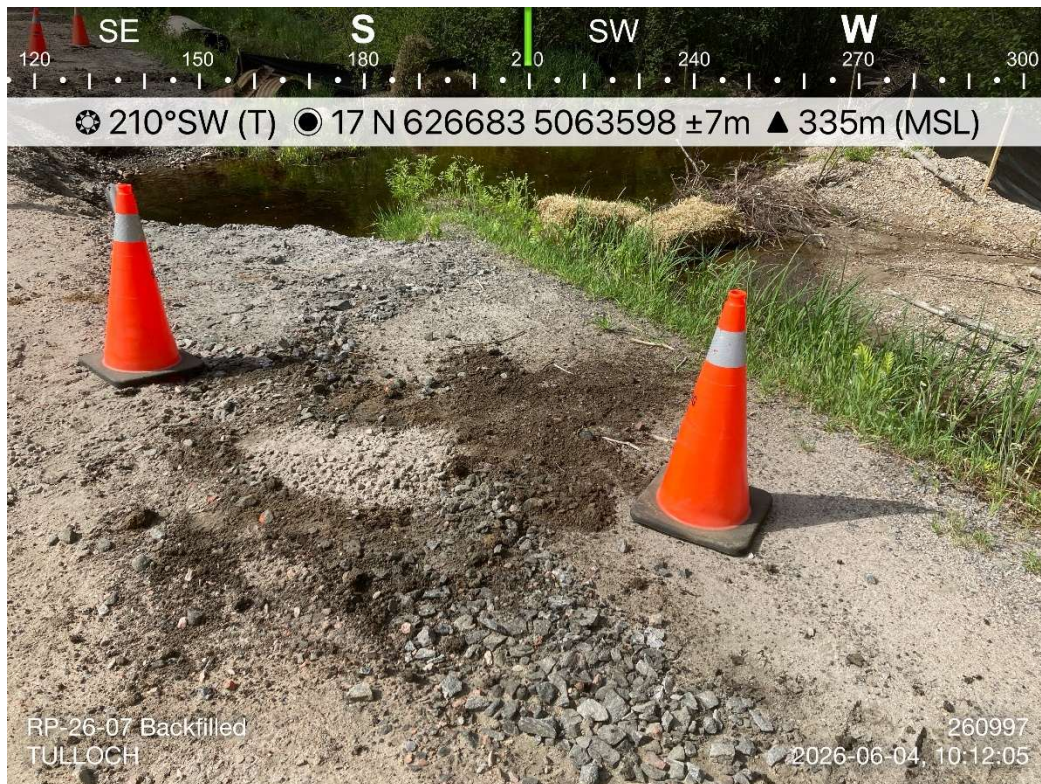
Photo 24: RP-26-07 Backfilled and Completed
