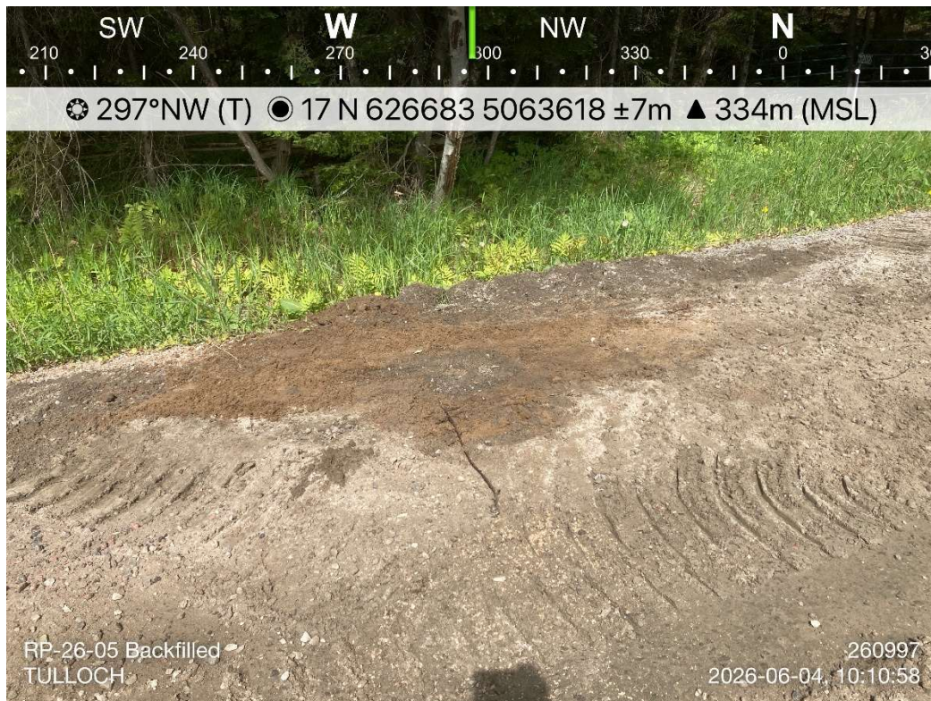
Photo 20: RP-26-05 Backfilled and Completed
