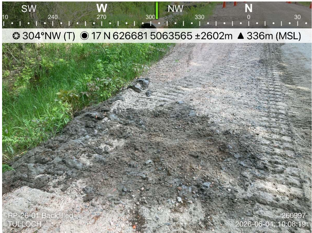
Photo 12: RP-26-01 Backfilled and Completed
