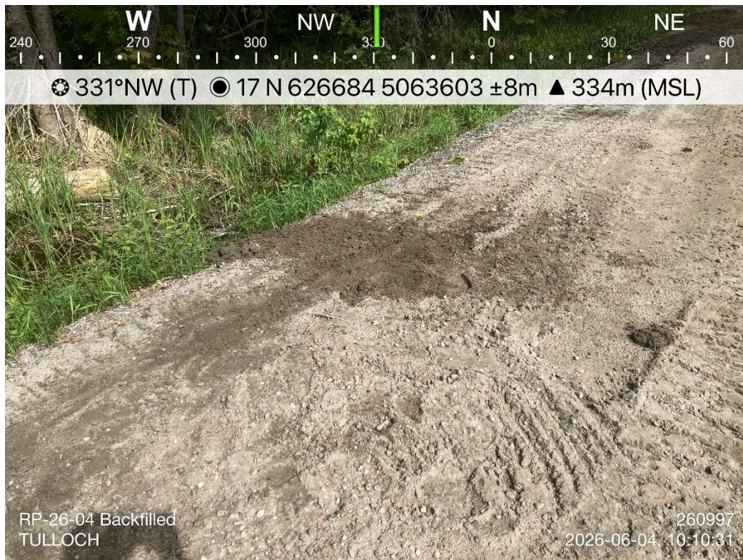
Photo 18: RP-26-04 Backfilled and Completed
