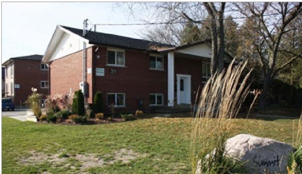
78 Stanley Avenue - Kitchener ON N2K 2B2
