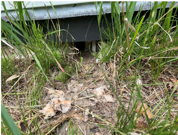
Exterior of Building:
